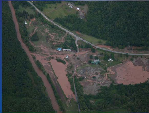
Aerial photograph of lower Spring Brook. Courtesy of Delaware County.
