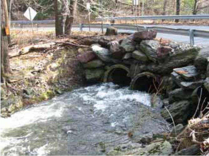
**Figure 7 - Cranberry Creek at Browns Hill Road: culvert is undersized, threatens road. Culvert should be replaced and sized sufficiently to provide additional cross sectional area and improve fish passage.**
