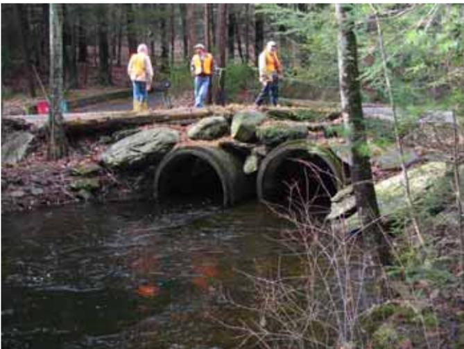
**Figure 8 - Cranberry Creek at Cranberry Creek Road crossing. Culvert undersized, road frequently floods. Stream receives a large amount of road runoff. Non-point source pollution management recommended here.**
