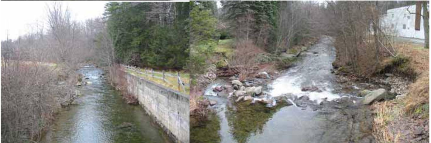
**Figure 20 – Upper Paradise Project 2: Pocono Gardens Resort Site – upstream view of channelized section (above) and downstream view past breached dam (right).**
