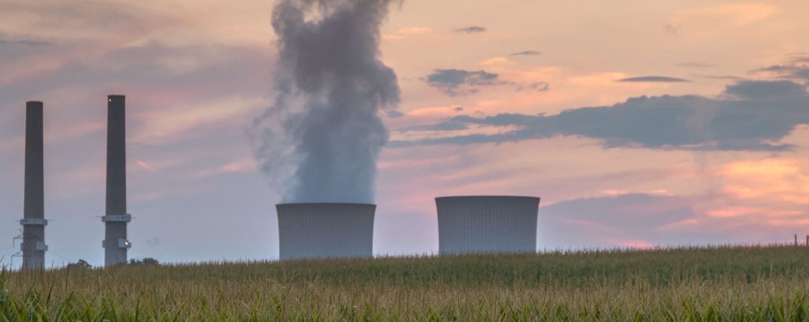
A natural draft cooling tower visibly shows a portion of withdrawn water not being returned (evaporation). Photo © Cheryl Fleishman | Dreamstime
