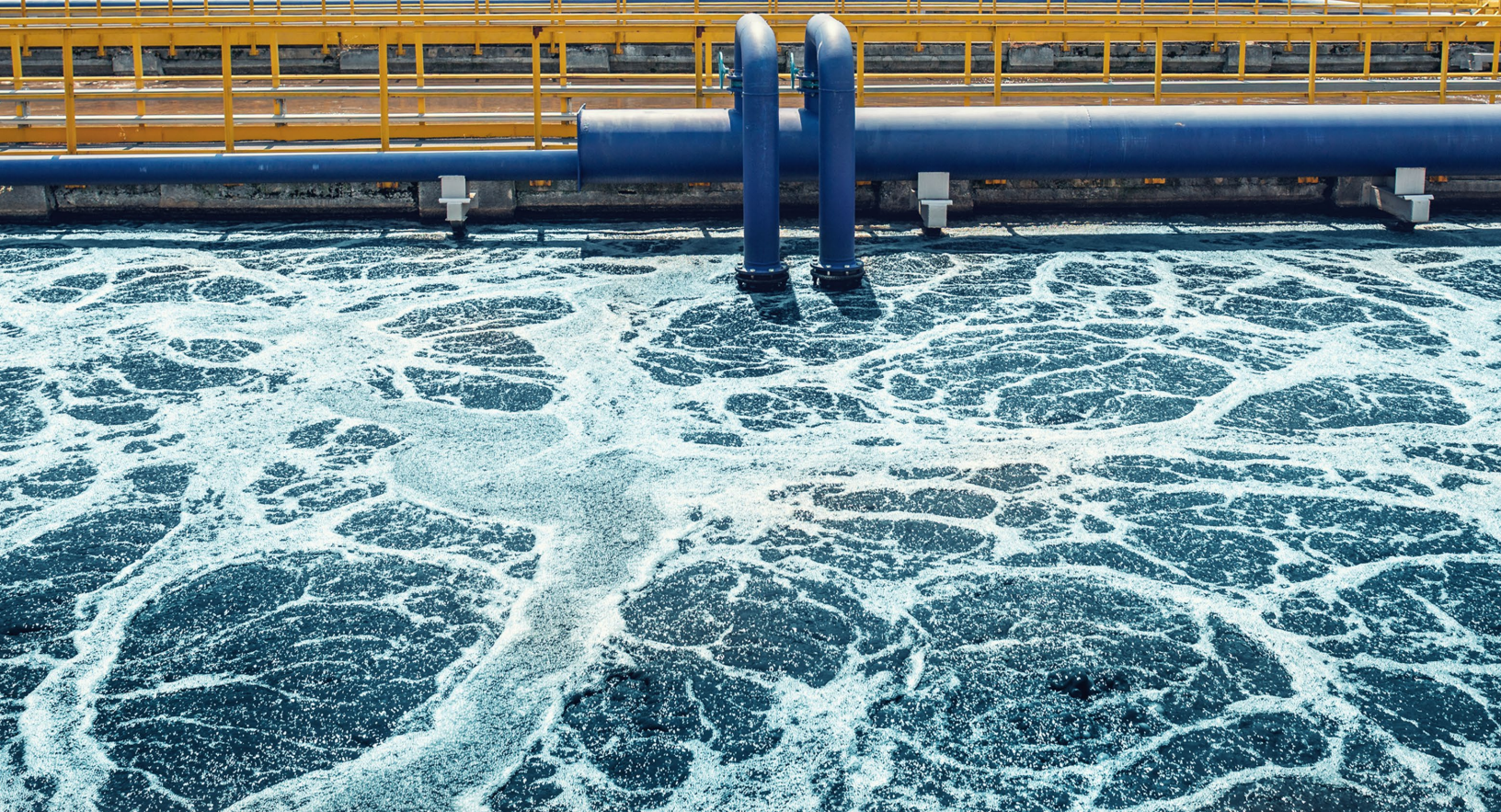
Wastewater treatment plants aerate wastewater to raise dissolved oxygen levels. Photo © Dedmityay | Dreamstime
