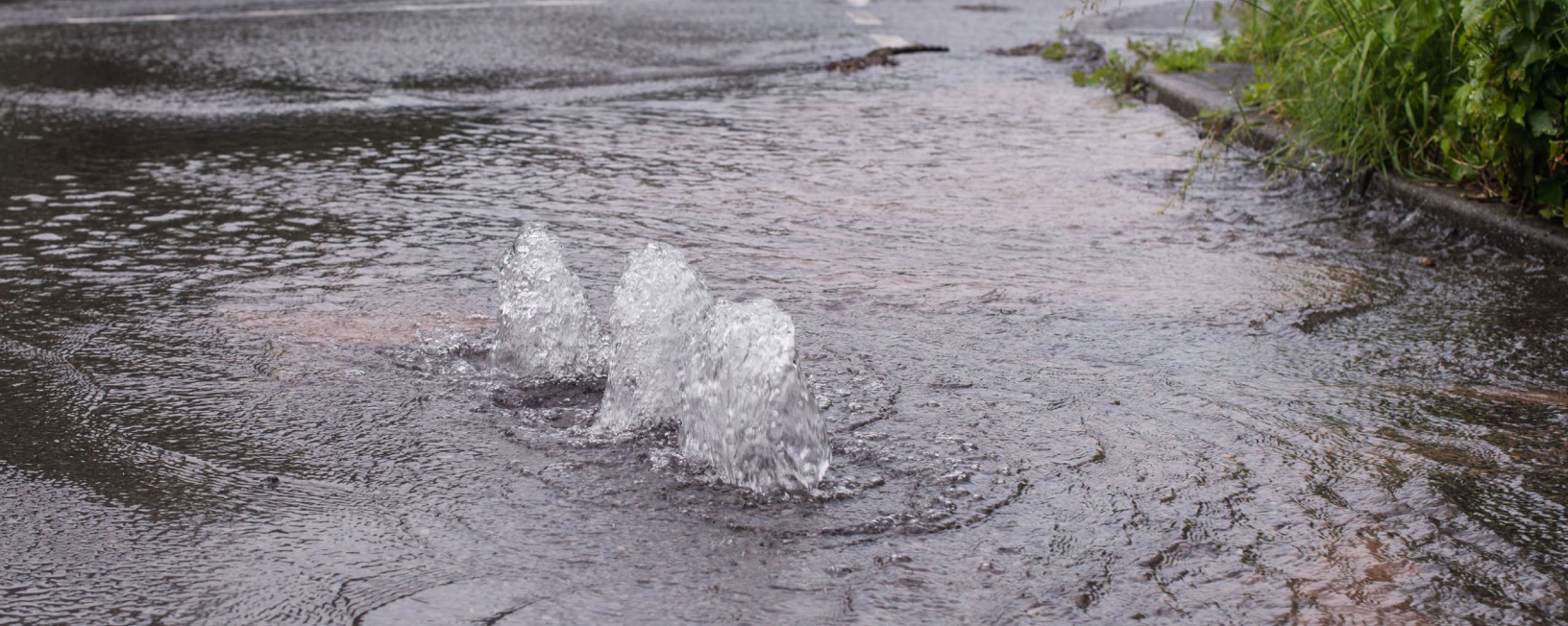
A burst underground water main results in visible leakage (real losses). Photo © Nigel Spooner | Dreamstime
