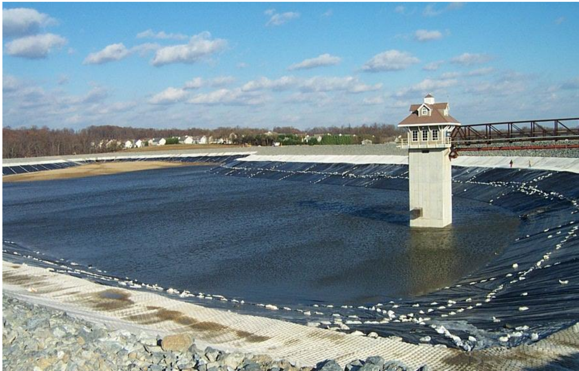
Newark Reservoir filling with geomembrane, concrete, and rock liner system (Dec 2005)
