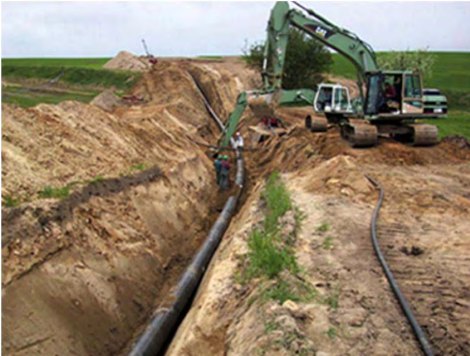
Fiber Optic Cable
