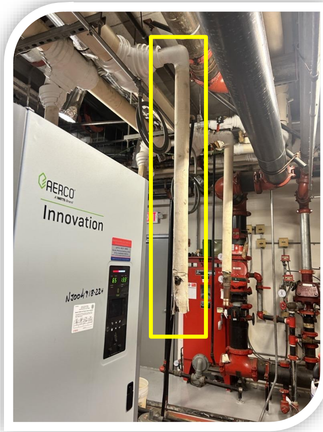
Respond to Hazardous Conditions Noted During the Risk Assessment (e.g., Assess the Water System for Dead Legs)
