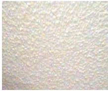
Trowelled on asbestos
