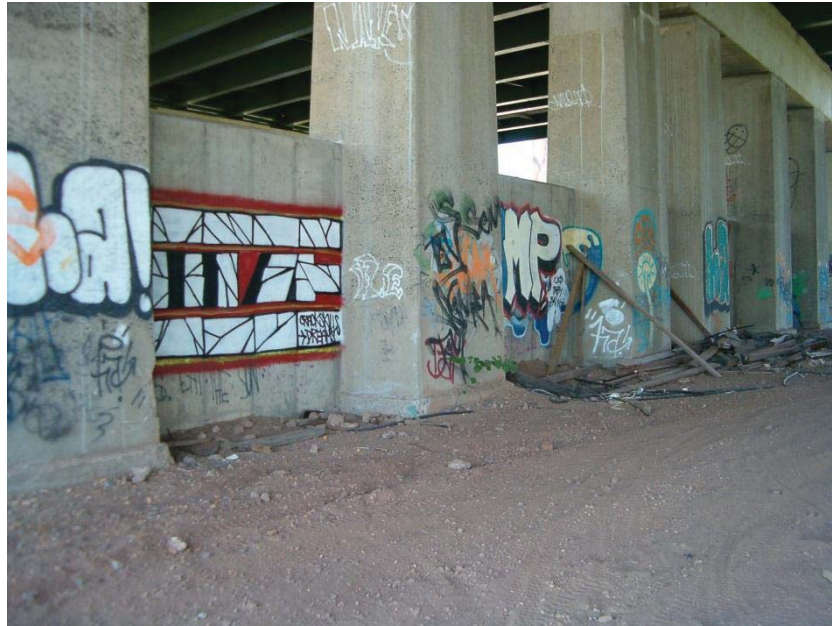
Photograph 5: Accessible areas under bridge
