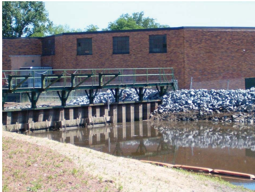
Photograph 6: Tide gate on Berry's Creek
