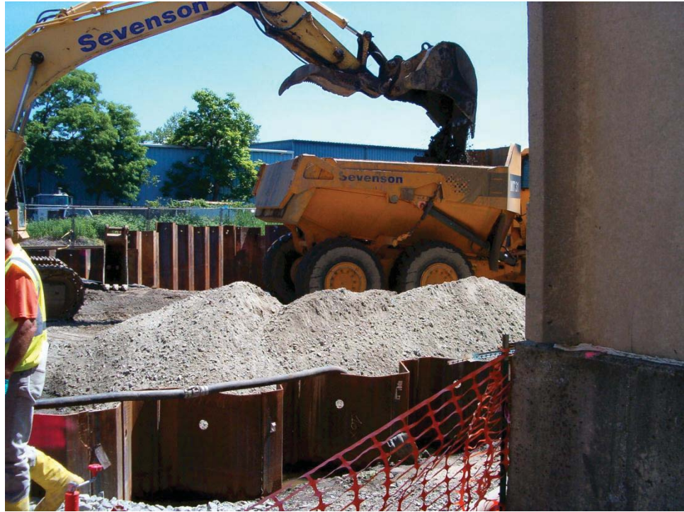
Photograph 1: Excavation of contaminated soil
