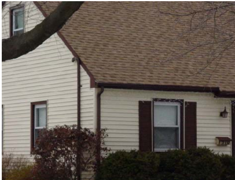
Photograph 2: Ventilation System installed at a residential building
