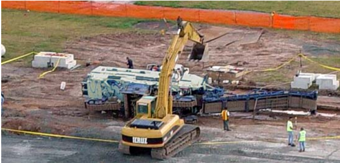
Photo 2 Photo of incident site showing excavator lifting machine (Port Authority Police)
