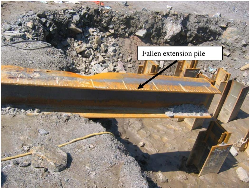
Figure 3: Fallen extension pile.
