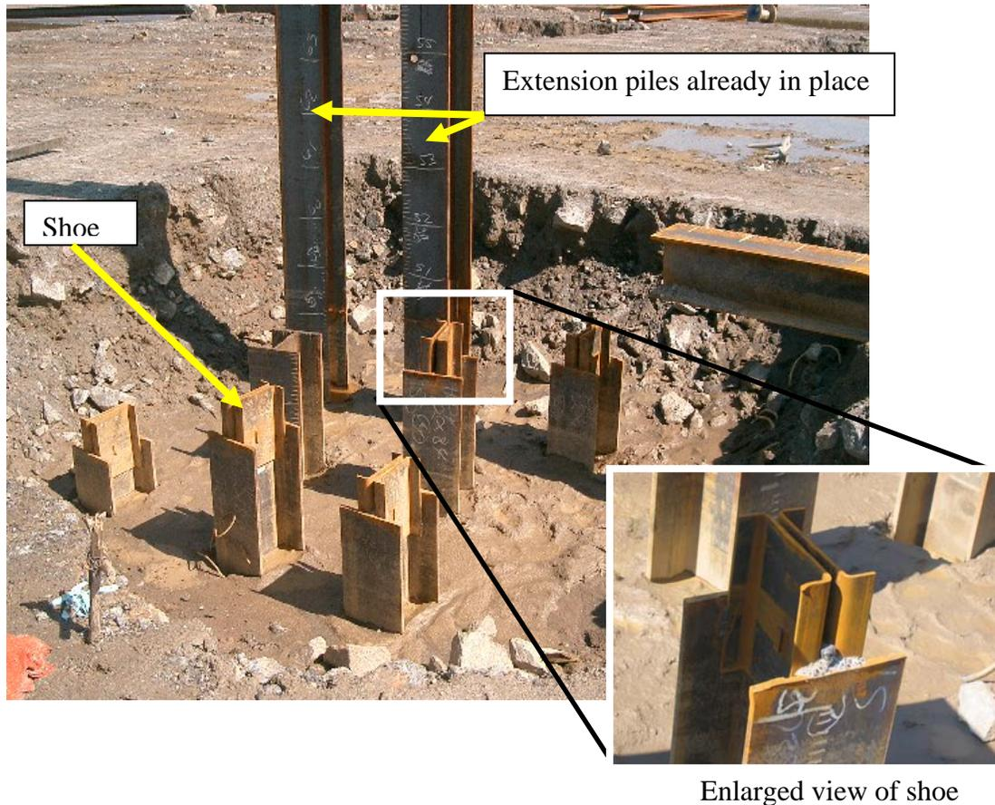
The incident occurred at approximately 9:45 AM on Tuesday, August 29, 2006, a damp and rainy day. The job started at 7:00 AM, and a crew of four began “knitting” (welding) extension piles to the first of eight to be completed in the pit on that day; no hammering was to be done on this day. Just prior to the 9:15 AM break, the crew successfully knitted the second extension pile. Work resumed at approximately 9:30 AM, and the incident occurred shortly thereafter.
