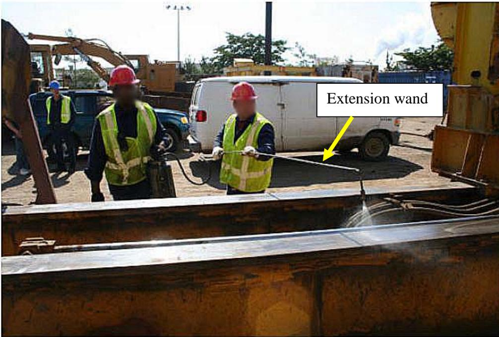
NJ FACE also recommends that the control of hazardous energy should be considered. According to 29 CFR 1917.151(b)(7) (*Marine Terminals, Related Terminal Operations and equipment*): The power supply to machines shall be turned off, locked out, and tagged out during repair, adjustment or servicing. Therefore, the container spreader should be de-energized while being lubricated.<sup>1</sup>
