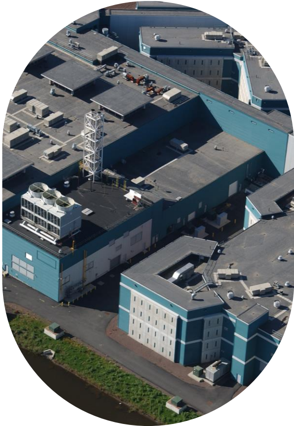
Photo of Essex County Correctional Facility
