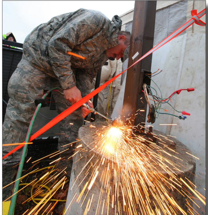
Staff Sgt. Carl Hilpl, 108th Wing, New Jersey Air National Guard, cuts the bolts holding a light pole at the Ocean County Medical Center in Brick, N.J., Nov. 7, 2012. More than 2,000 Airmen and Soldiers from the New Jersey National Guard have been mobilized in response to Hurricane Sandy.
