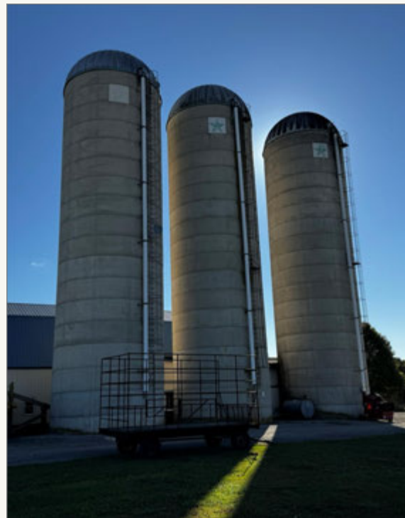
Silos at Riverside Greenhouses, Allamuchy Township
