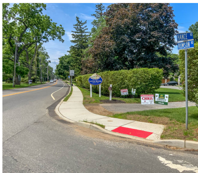
Little Silver Borough Sidewalk Repair. SFY2022 Loan: $2,388,507
