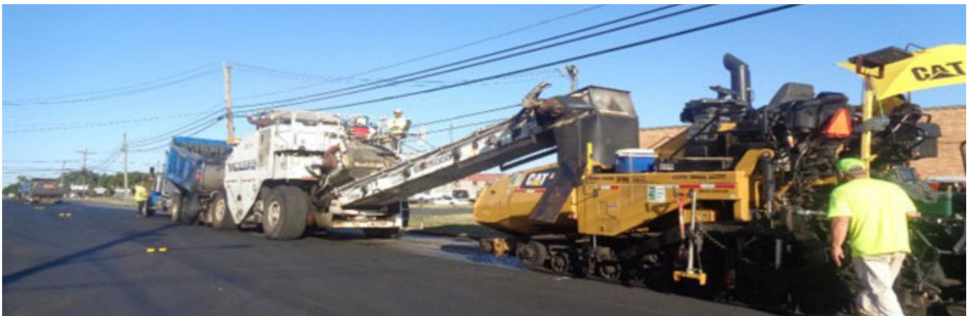
Camden County Westfield Avenue Reconstruction. SFY2022 Loan: $1,786,364
