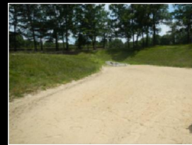
Newly constructed K5 sand lined basins
