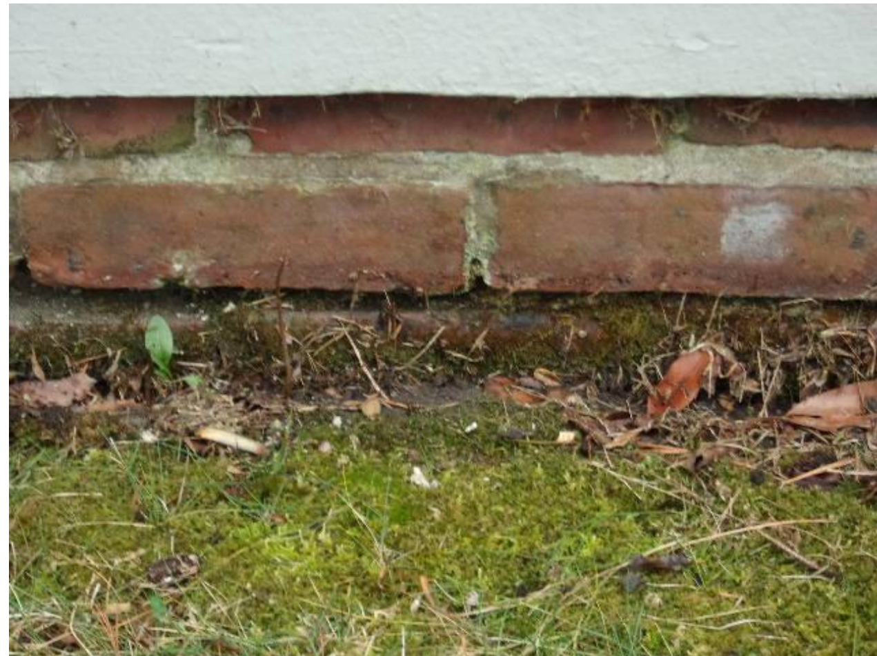
Brick foundation mortar repair
