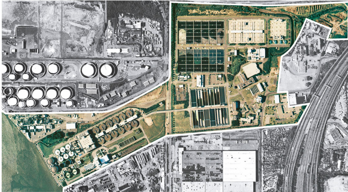
Aerial View of the Passaic Valley Sewerage Commission Facility
