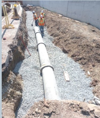
Images (clockwise from the top): The interior of the floodwall along Wilson Avenue; an automatic, heavy-duty gate being installed near the intersection of Avenue P and Rutherford Street; work being performed on one of PVSC's pump station wet-wells; drainage piping for PVSC's floodwater collection system being installed.
