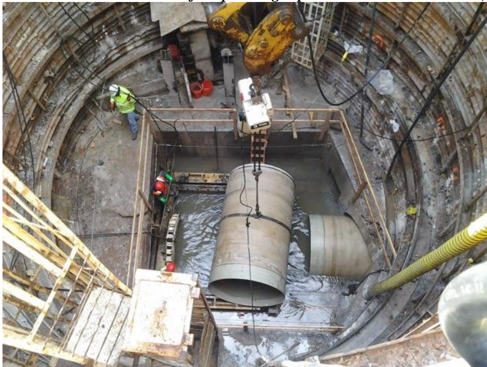
Photograph No. 08 – Scribner Place Access Shaft Slip-Lining Pipe Installed towards MH MI-145 (Hamilton Avenue).
