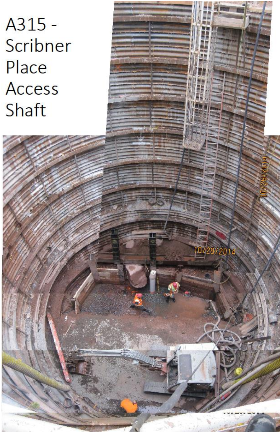
Photograph No. 04 – Scribner Place Access Shaft (within public right-of-way) between Clifton Avenue and Mahr Avenue – Significant Bedrock and Groundwater Encountered During Excavation. [Approximately 28-feet deep]
