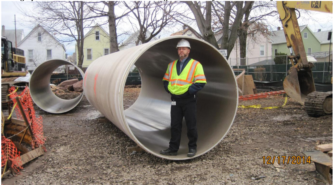
Photograph No. 06 – Perspective Point of View of the Size of the Slip-Lined Pipe (72-Inch Diameter).
