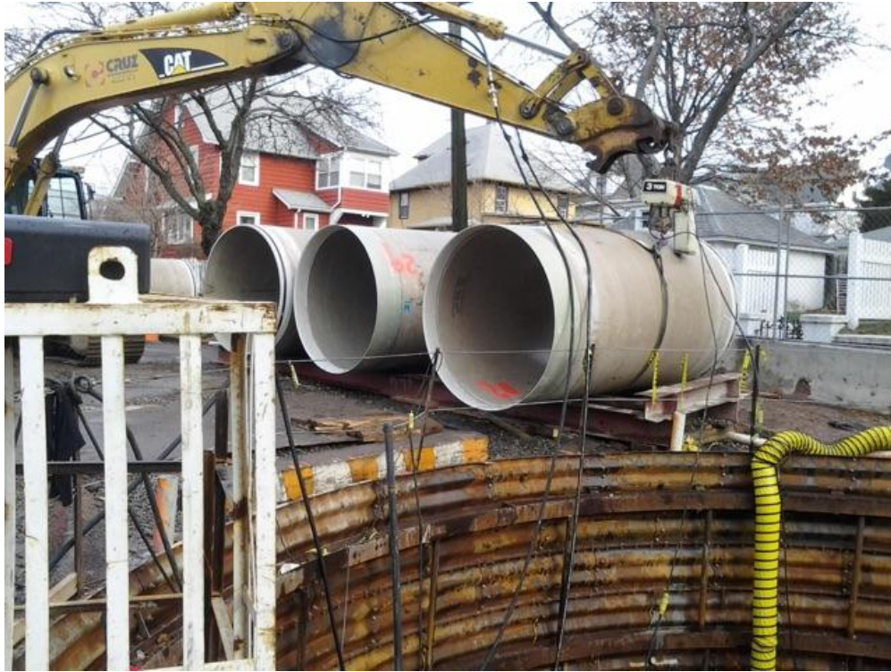
Photograph No. 09 – Scribner Place Access Shaft Slip-Lining Pipe Staging Area.
