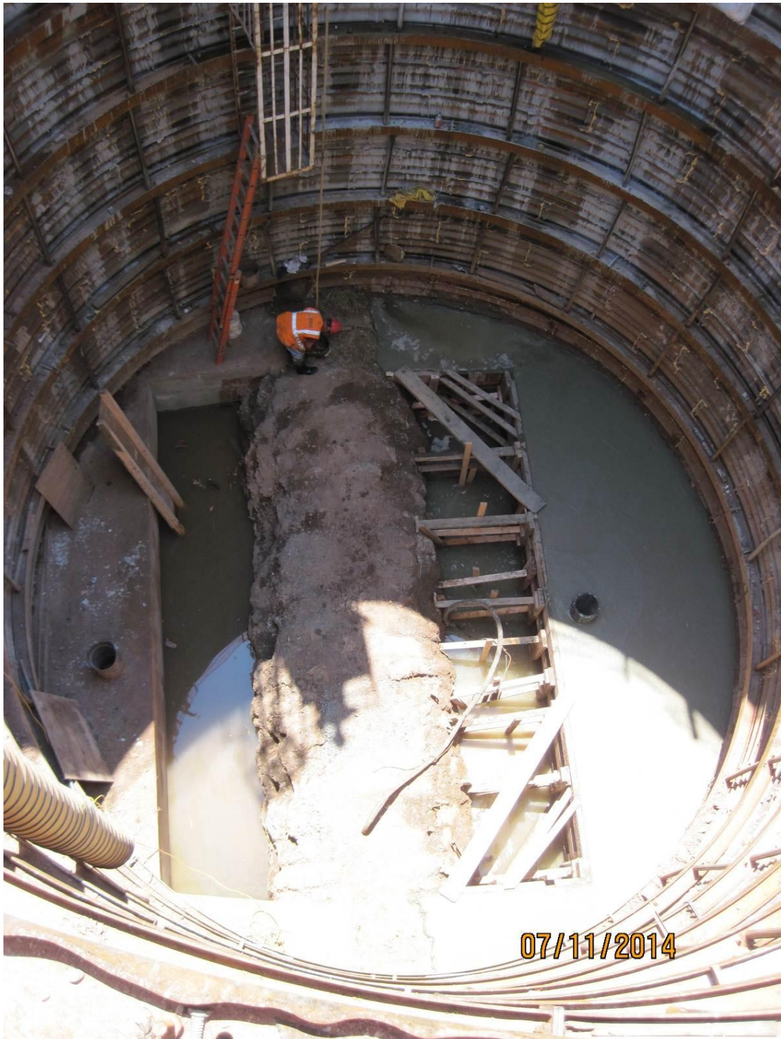
Photograph No. 03 – Cutler Street Access Shaft (within private property) – Significant Bedrock Encountered During Excavation. [Approximately 31-feet deep]
