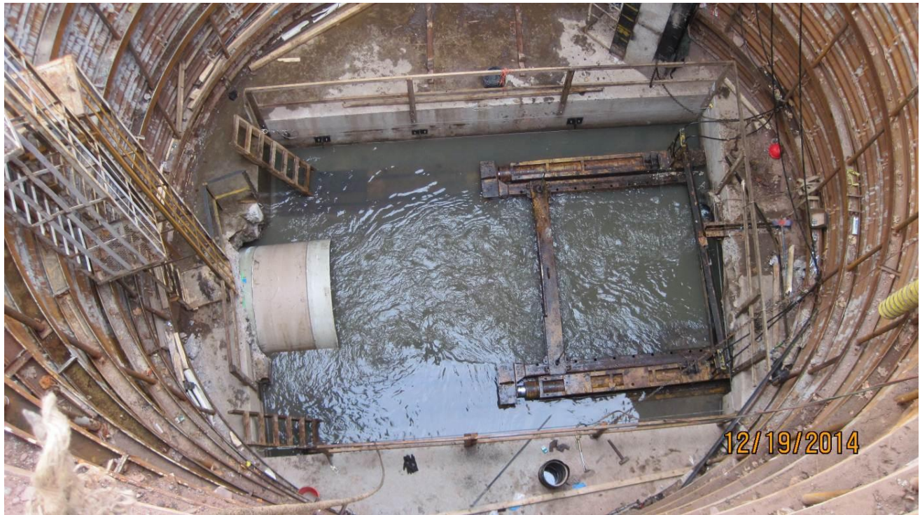
Photograph No. 07 – Cutler Street Access Shaft Slip-Lining Pipe Installed to MH MI-141 (Hope Avenue).
