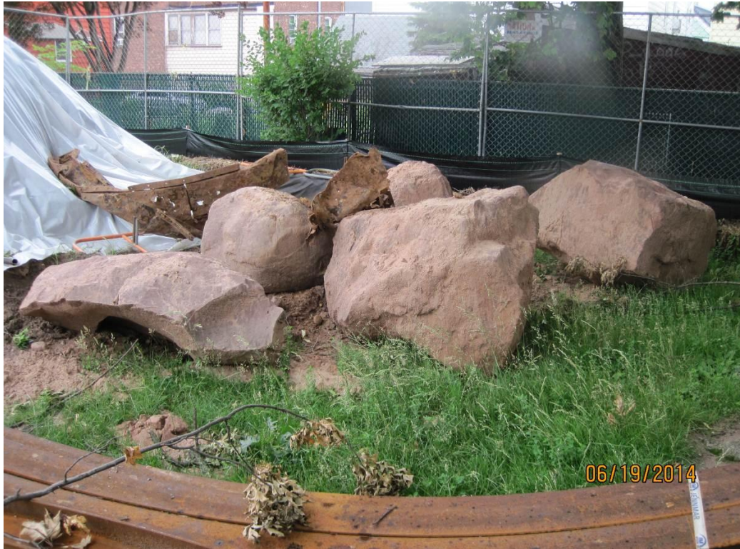
Photograph No. 05 – Bedrock Encountered during Excavation of both Access Shafts.
