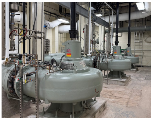
Images: The new vertical dry centrifugal pumps (left); and the new grinders/comminutors (right).
