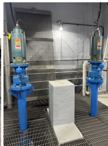
Images: The new vertical dry centrifugal pumps (left); and the new grinders/comminutors (right).
