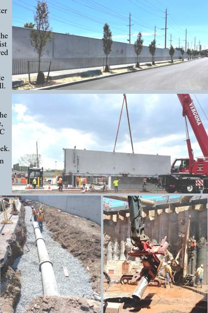
Images (clockwise from the top): The interior of the floodwall along Wilson Avenue; an automatic, heavy-duty gate being installed near the intersection of Avenue P and Rutherford Street; work being performed on one of PVSC's pump station wet-wells; drainage piping for PVSC's floodwater collection system being installed.
