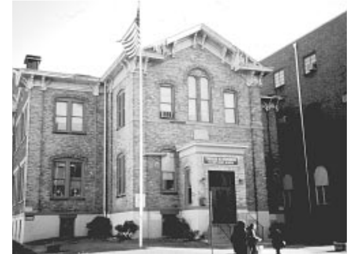
This old school building in Perth Amboy illustrates the opportunity to preserve an architecturally distinctive facility that is conveniently located to downtown neighborhoods.
