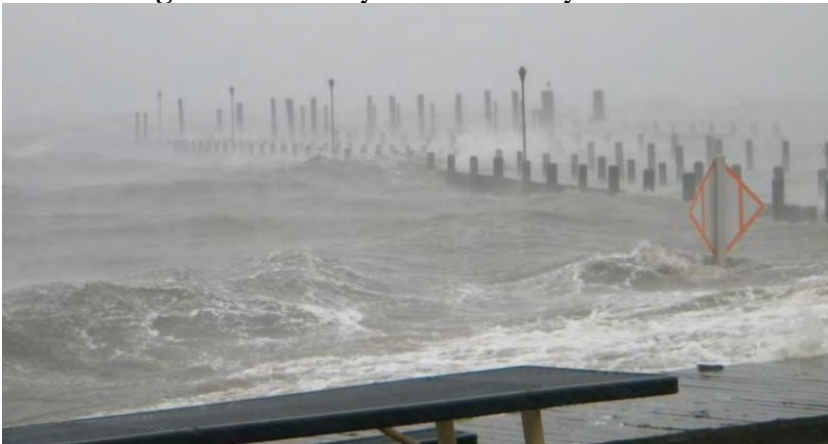
Figure 10: Destroyed Dock at Bryant Park
