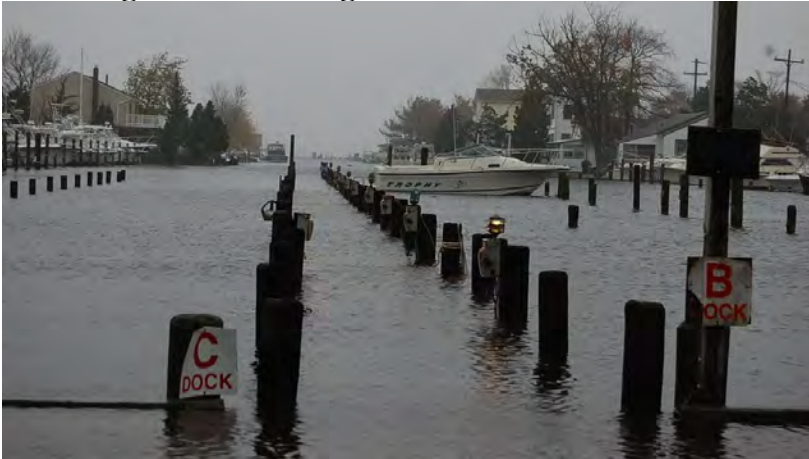
Figure 12: Flooding at the Tuscarora Park Area
