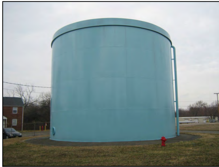
300,000-gallon ground water storage tank
