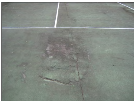
Worn and cracked playing surface
