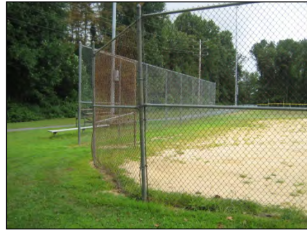
Rusty and warped back-stop
