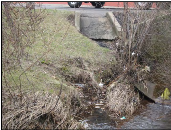
Storm water channel into the North Run from Fort Dix Street. Trash and debris are present.
