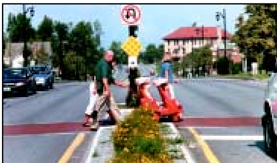
Figure 2.5: Conforming median, Burlington, Vermont.
