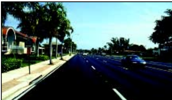
Figure 2.12: Edge lines with small offsets on Main Streets in Dublin, New Hampshire (top) and Deerfield Beach, Florida (bottom).
