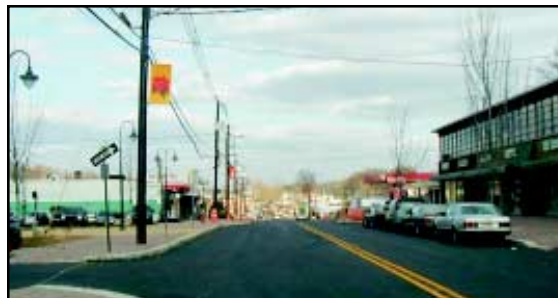
Figure 3.2.2.5: After at Train Station Plaza.
