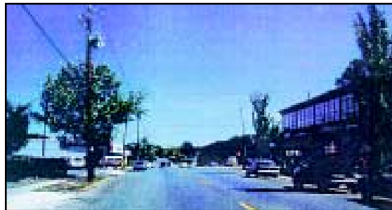
Figure 3.2.2.4: Before at Train Station Plaza.
