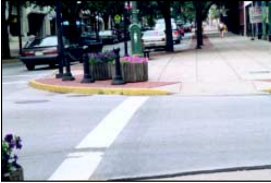
Figure 2.26: Twenty-foot corner with alternate truck route, York, Pennsylvania.
