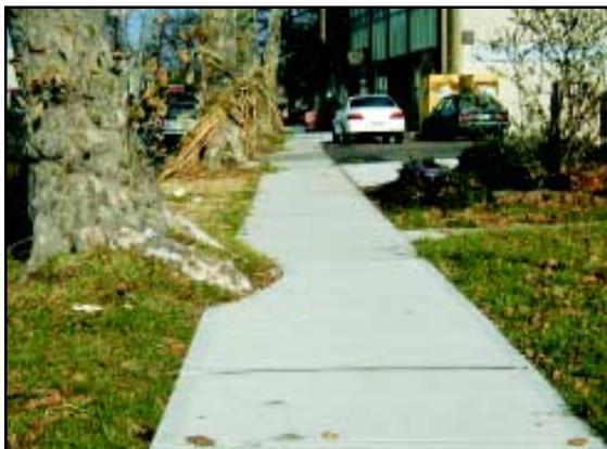
Figure 3.2.2.18: Sidewalk at tree.
