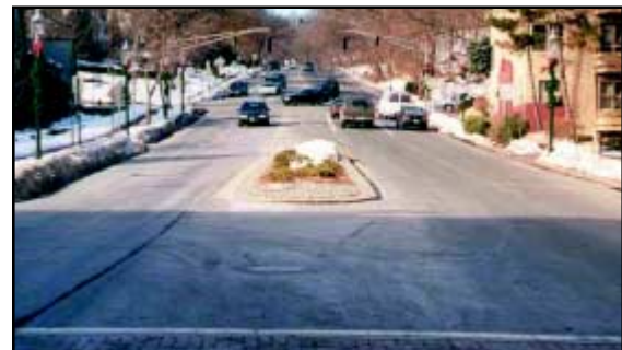
Figure 3.2.3.12 Raised median as a gateway into town.
