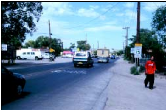
Figure A.2.2: Section of Isleta Boulevard requiring reconstruction, Albuquerque, New Mexico
