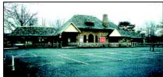
Figure 3.2.2.21: Former train station.
