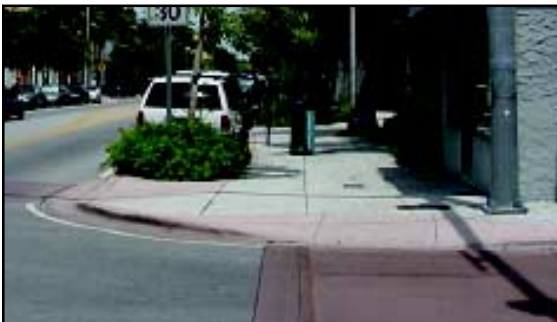
Figure 2.28: Fifteen-foot mountable corner, South Miami, Florida.
