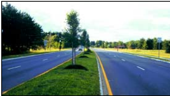
Figure 3.3.4.5: Twelve-foot raised median.
