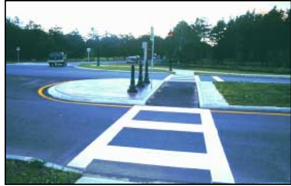
Figure 3.3.4.19: Well-marked crosswalk and accessible median.
