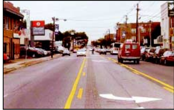
Figure 3.2.1.4: Former centerline, existing two-way left-turn lane.
