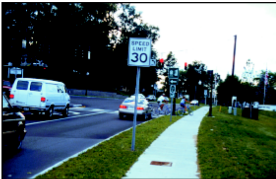
Figure 3.3.4.18: New sidewalk condition.
