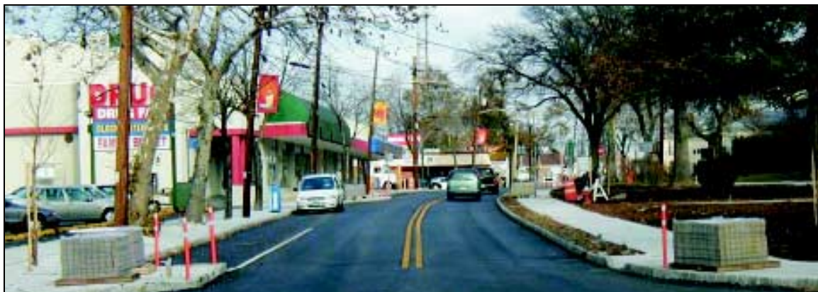
Figure 3.2.2.1: South Avenue construction.
