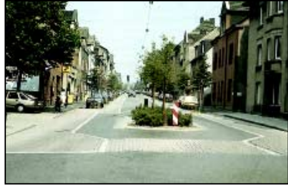
Figure 2.34: Traffic calmed main street in Recklinghausen, Germany.
