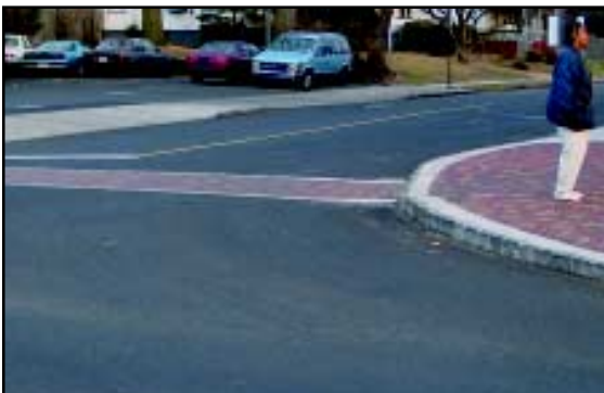
Figure 2.29: Twenty-foot corner with planned encroachment, Plainfield, New Jersey.
