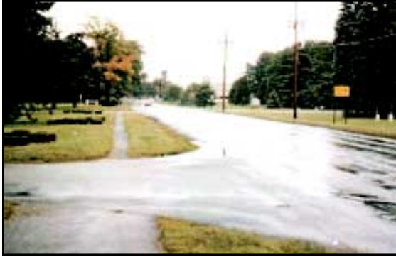
Figure 3.3.4.17: Former sidewalk condition.
