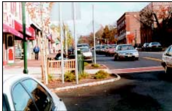
Figure 3.2.3.17 Curb extension narrows mid-block crossing.
