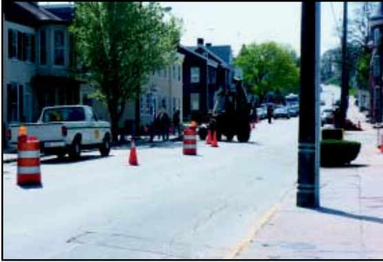
Figure A.2.4: East Main Street during reconstruction, Westminster, Maryland
