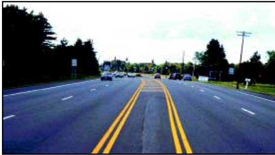
Figure 3.3.4.4: Twelve-foot flush median.
