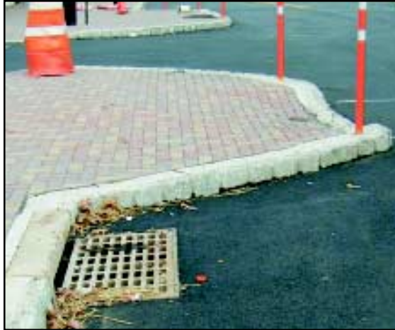
Figure 3.2.2.8: Inlet at curb extension.
