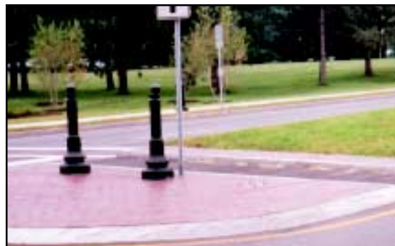
Figure 3.3.4.15: Missing bollard at Avenue of the Pines intersection.
