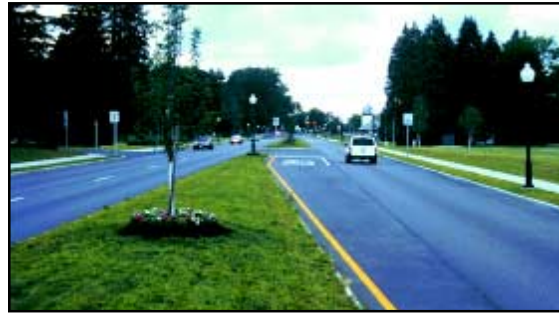
Figure 3.3.4.7: Twenty-three foot raised median with turn bays.
