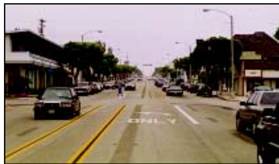
Figure 2.6: Nonconforming median, Los Angeles, California.
