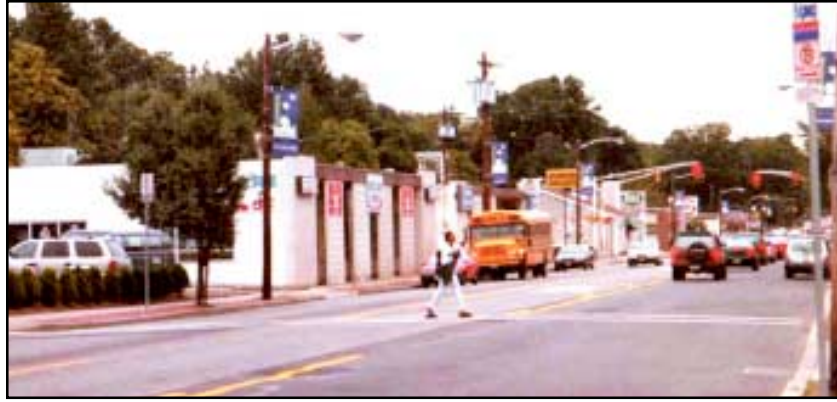
Figure 3.2.1.13: Existing uncontrolled crosswalk.
