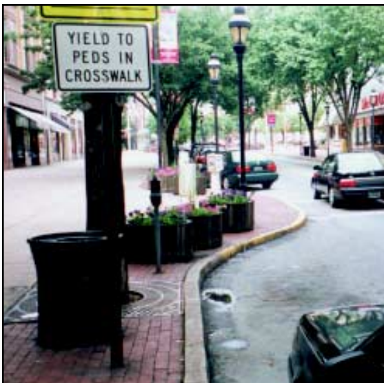
Figure 3.3.6.21: Curb extension and signage at mid-block crosswalk.
