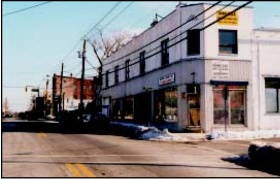
Figure 3.2.1.8: Existing at Ohio Street.
