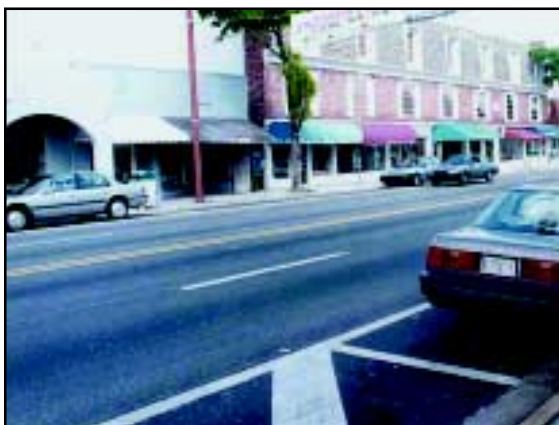
Figure A.2.8: Sunset Drive before reconstruction, South Miami, Florida.
