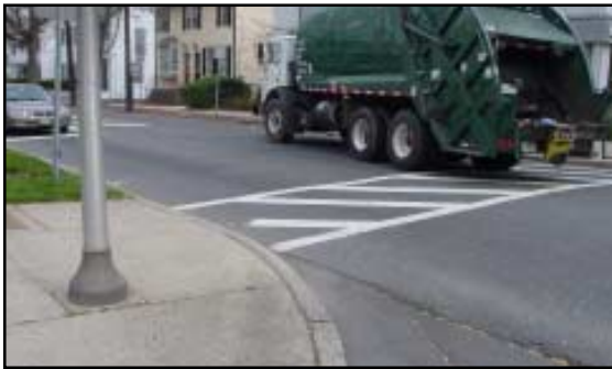
Figure 2.31: Fifteen-foot corner with stop lines set back, Princeton, New Jersey.
