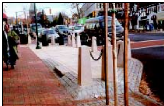
Figure 3.2.3.18 Curb extension with bollards.
