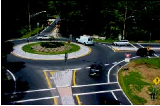
Figure 3.3.3.11: New roundabout between Sag Harbor and North Haven.
