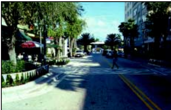
Figure 2.19: Curb extensions at a midblock crossing, West Palm Beach, Florida.
