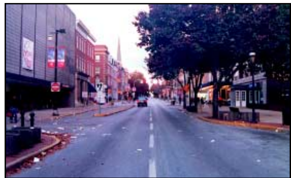
Figure 3.3.6.15: Market Street at parking garage (contra-flow lane).
