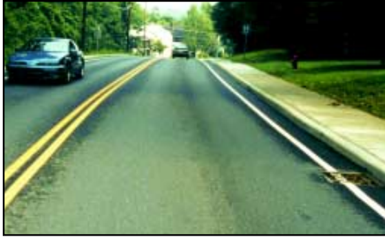
Figure 3.3.1.5: Drainage grate and edge line.
