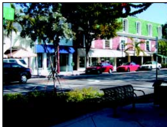
Figure A.2.9: Sunset Drive after reconstruction, South Miami, Florida.
