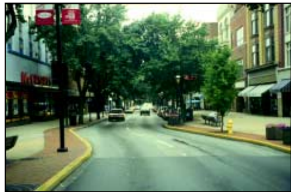
Figure 2.35: Traffic calmed main street in York, Pennsylvania.
