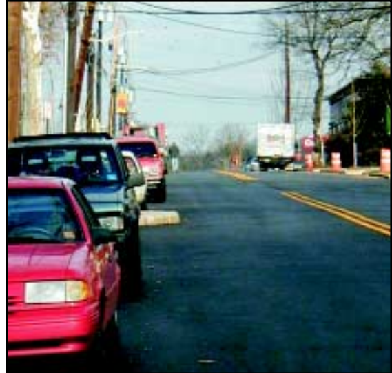
Figure 3.2.2.9: Curb extension poking out between parked cars.
