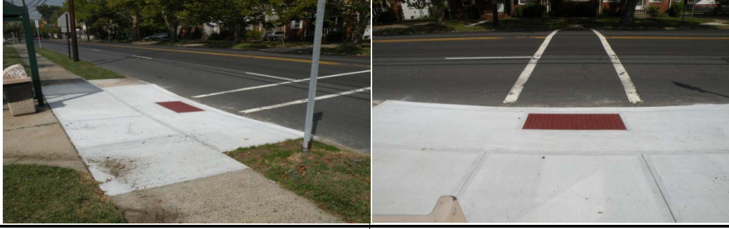
AFTER: Installed Curb Ramp at bus stop in front of MOB on Parkway Avenue, 9/3/10.
