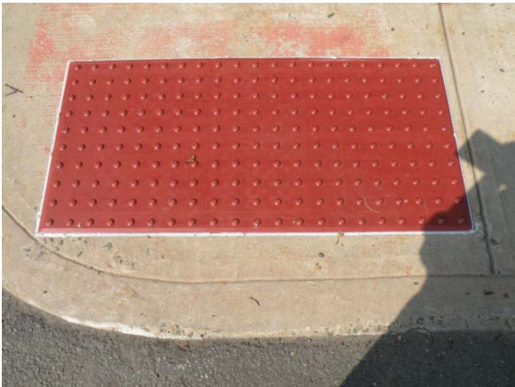
AFTER: Truncated Dome installed on 9/3/10
