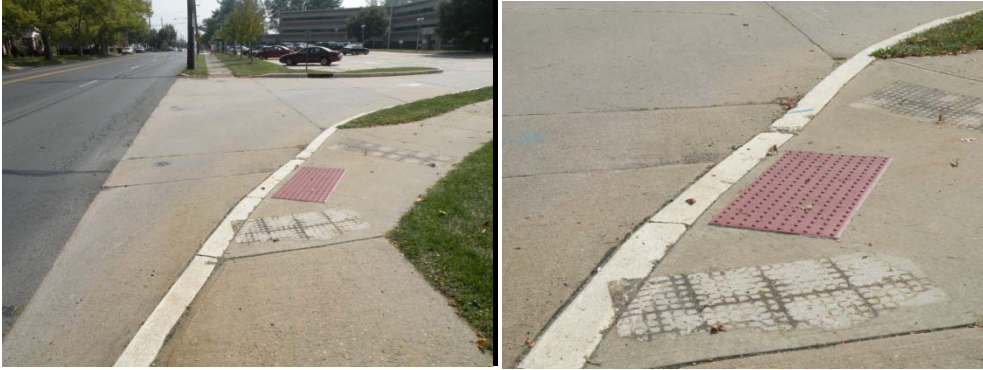
AFTER: Curb Ramps repaired and Truncated Domes installed on 9/3/10
