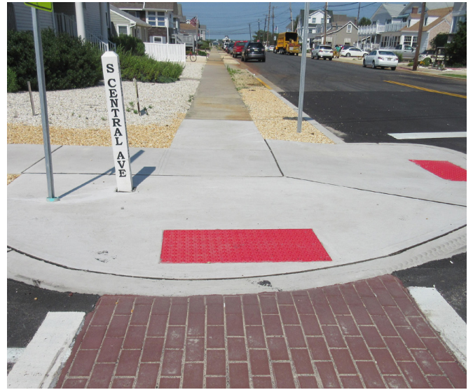
ROUTE 35 PAVEMENT RECONSTRUCTION
