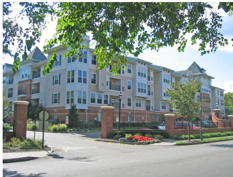
New housing in South Orange (Gaslight Commons) is designed
