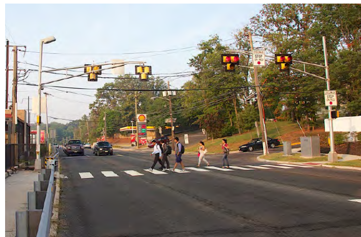
An NJDOT study found that motorists were much more likely to stop for pedestrians following the installation of this hybrid beacon on Route 27 in Woodbridge.
