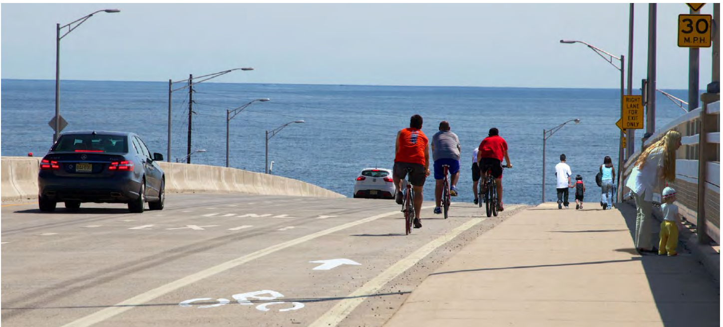
Bridge with bike lane in Highlands, NJ
