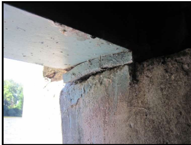
Figure C.1.2.4-1 – South Fascia Elastomeric Bearing
