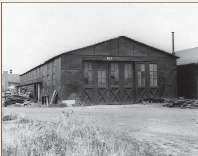
Building #4, Paint Shop, Built Circa 1924 (no longer extant). Photograph dates to 1949.
