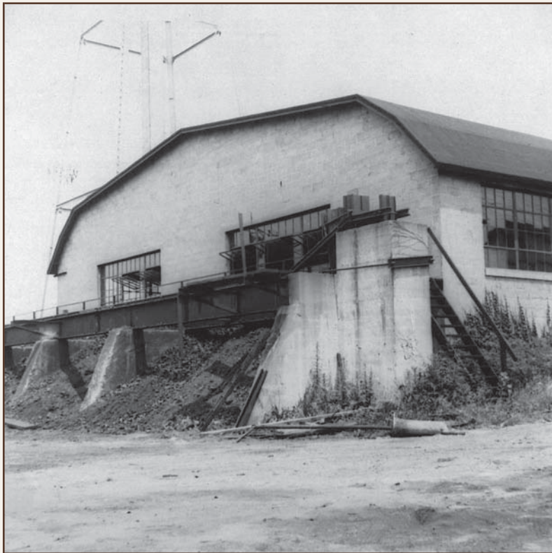
Building #2, Built in 1923. Looking north at rear. Note the elevated railroad track where cars could dump bulk materials into concrete bunkers. Photograph dates to 1949.
