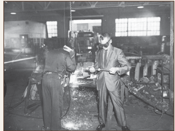
Welding Safety Inspection at Fernwood, 1971. The inspector (right), identified as George Rightmire, is checking for dangerous gases, while the welder (left), identified as Fred Mason, works.
