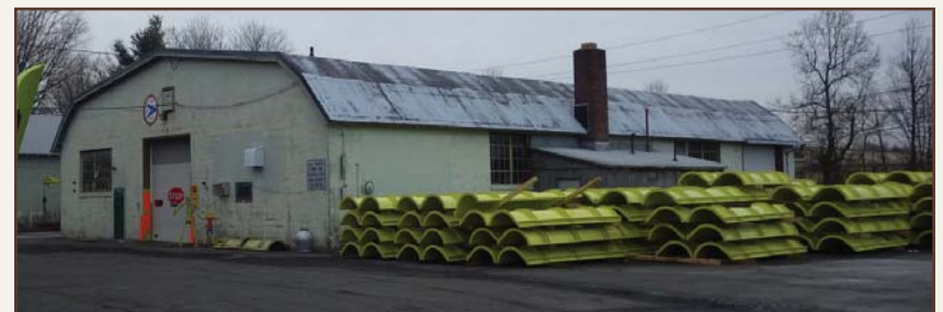
Building #2, Plow Shop, 2014.
