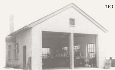
Building #25, Grease House, Built Circa 1940. Photograph dates to 1949.
