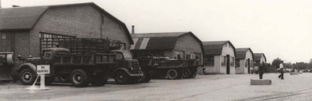
Building #s 7, 8, 11, 17 and 20 (left to right), 1949.
