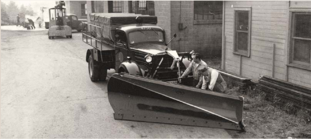
Attaching Plow to Truck for Snow Removal, 1950.
