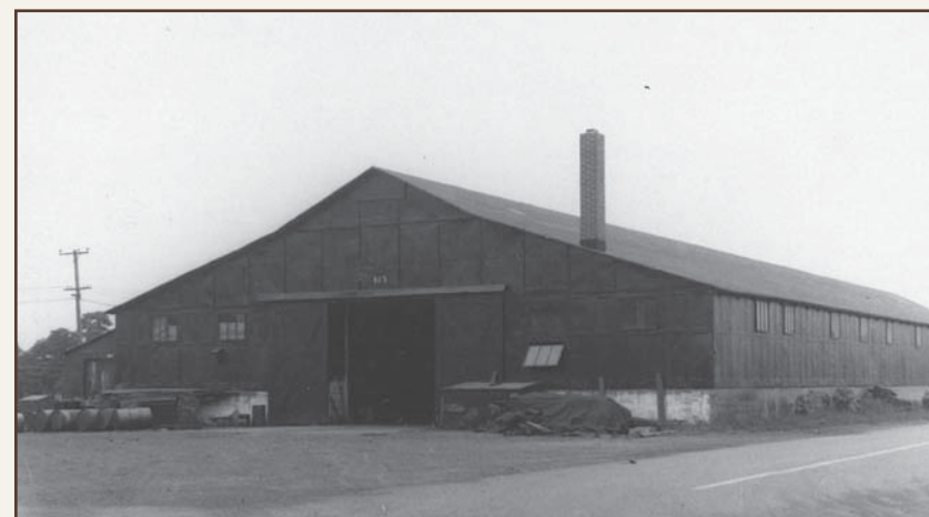
Building #5, Storage Building. View looking northwest. A prefabricated "Truscon" building, it was acquired as army surplus about 1925. Photograph dates from 1949.
