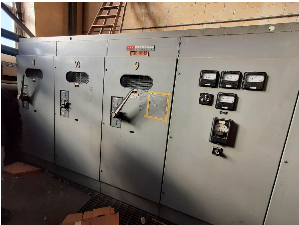
4800V Switchgear Lineup in the Powerhouse.
