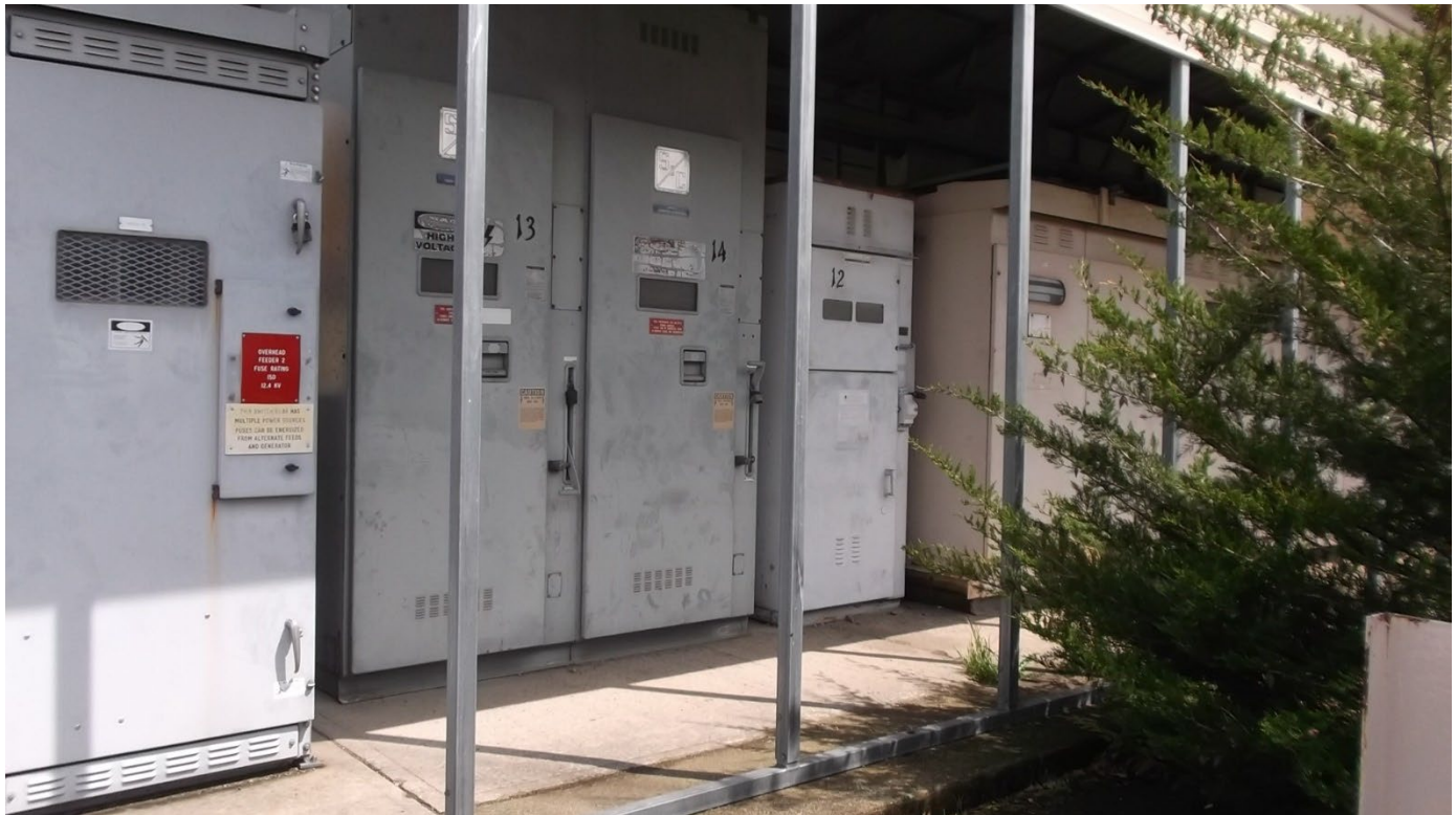
Main 12.47kV Switchgear Lineup outside of the Powerhouse at EMCF.
