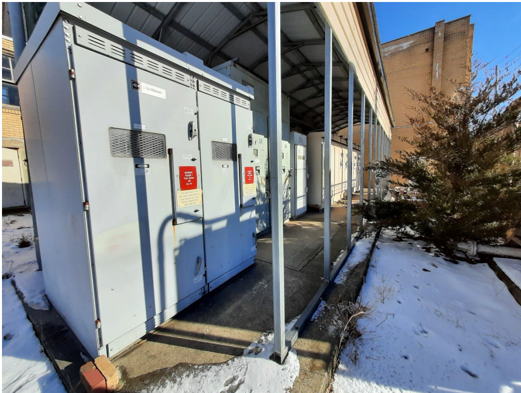
Main 12.47kV Switchgear Lineup outside of the Powerhouse at EMCF.
