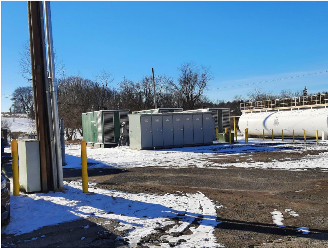
Fuel tank in background with fill port on wrong side.
