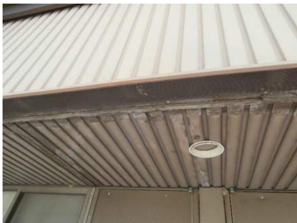
Figure 3.4 Metal soffit ceiling
