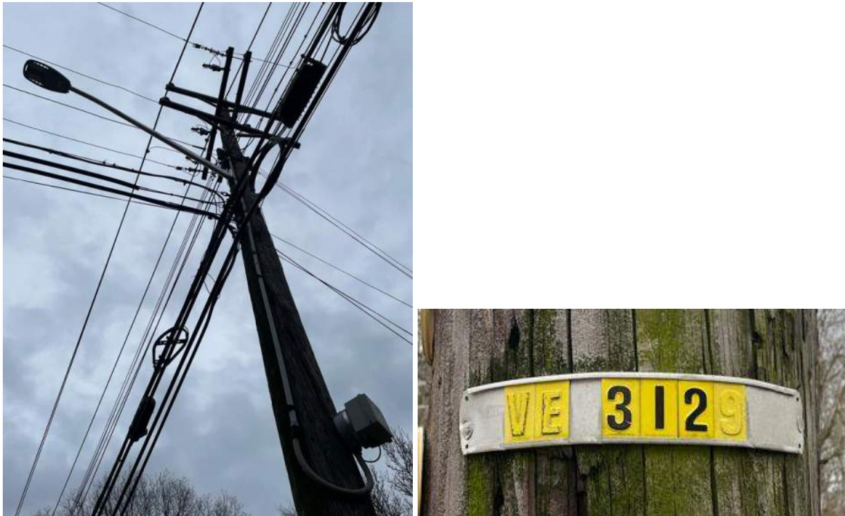
Figure 5.1 - Utility Pole #VE 3129
