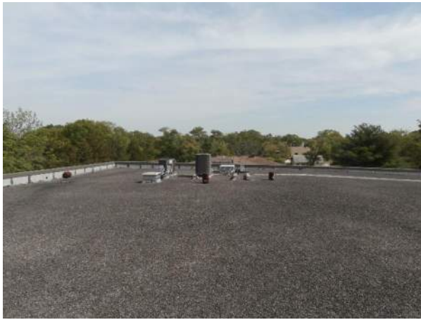
Figure 3.7 Typical flat built up roof
