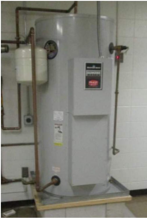
Figure 6.9 - Electric Water Heater
