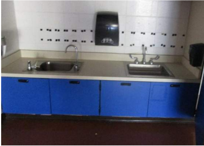
Figure 6.5 - Plumbing Fixtures, Sinks
