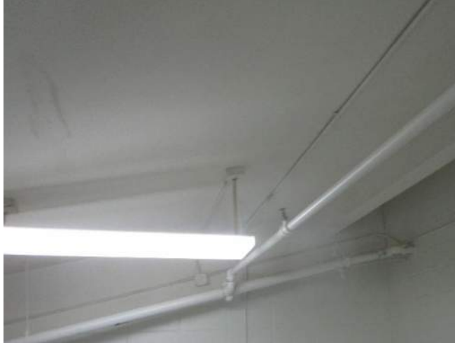
Figure 7.3 - Sprinkler Piping
