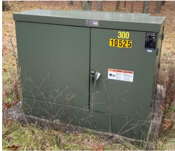
Figure 5.2 - 300kVA Transformer
