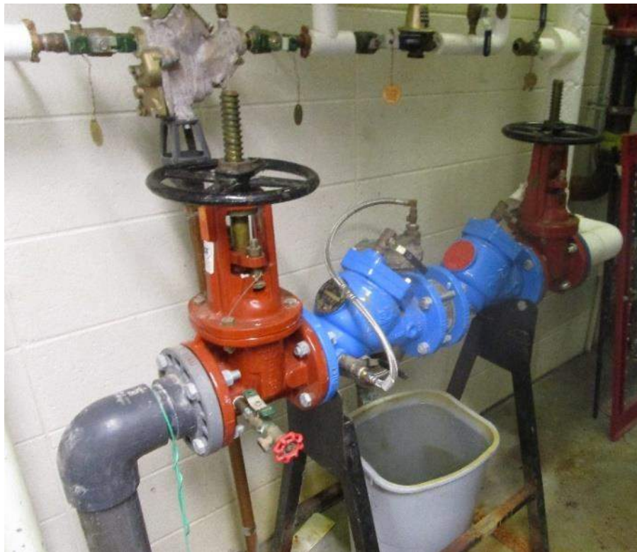
Figure 6.1 - PRZ Backflow Preventer
