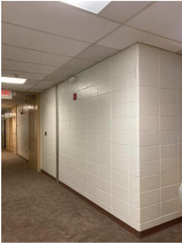
Figure 3.11 Typical CMU wall
