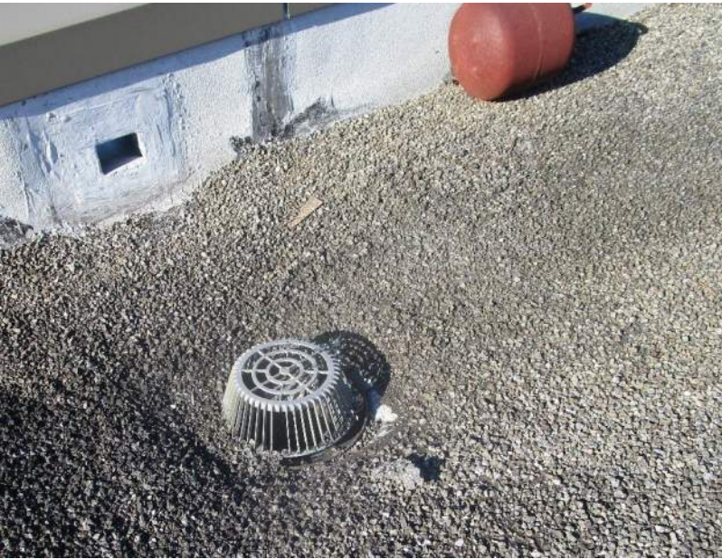
Figure 6.11 - Roof Drain
