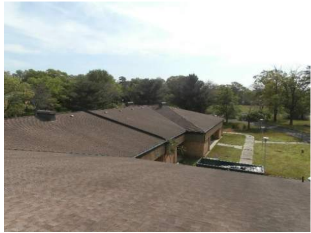
Figure 3.8 Typical shingle roof
