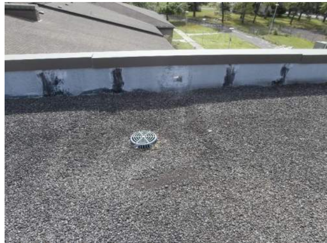
Figure 3.10 Typical roof drain and overflow
