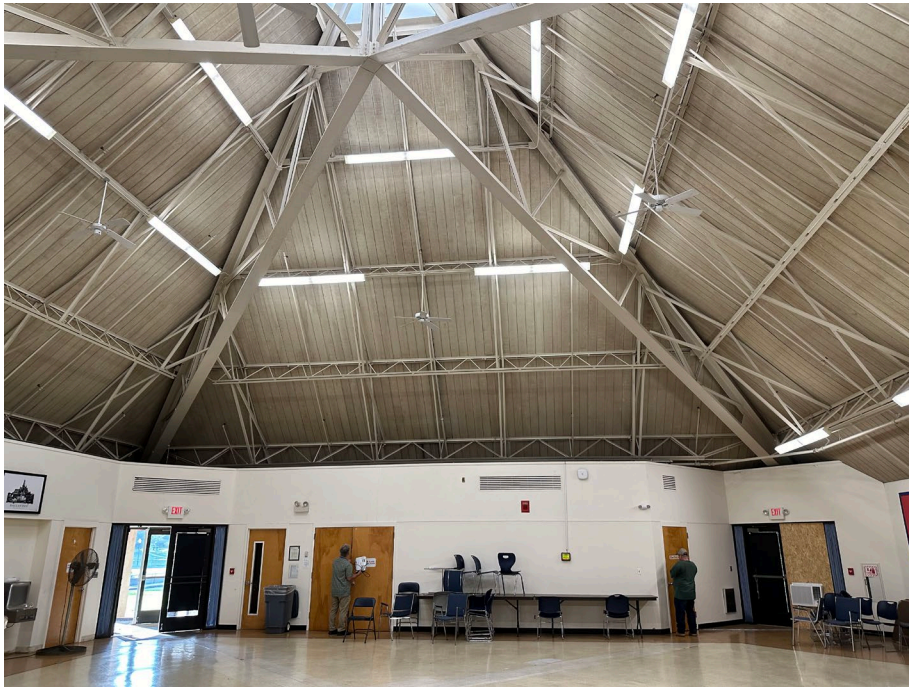
Existing Supply Grilles in Main Room
