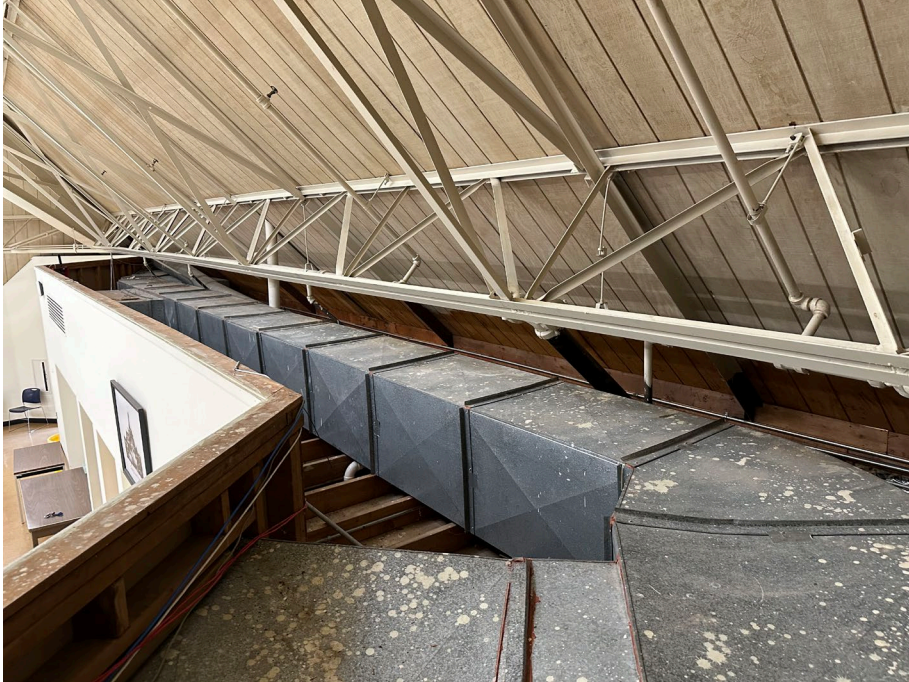
Existing Ductwork above rooms
