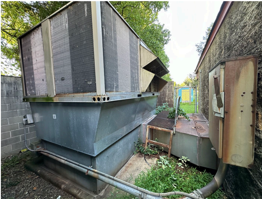
Existing Roof Top Unit
