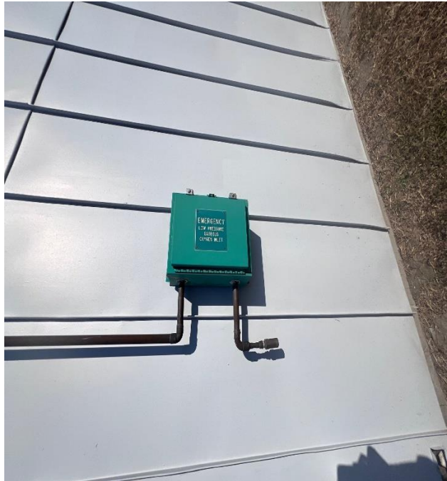
OXYGEN INLET LOCATION
