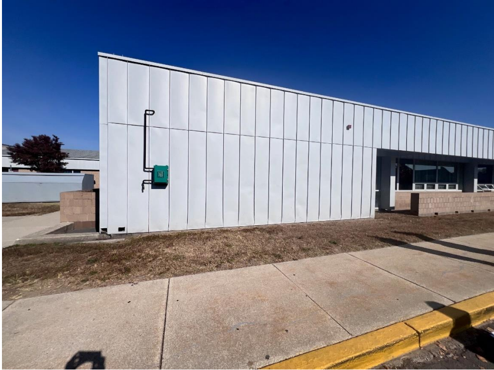
OXYGEN INLET LOCATION
