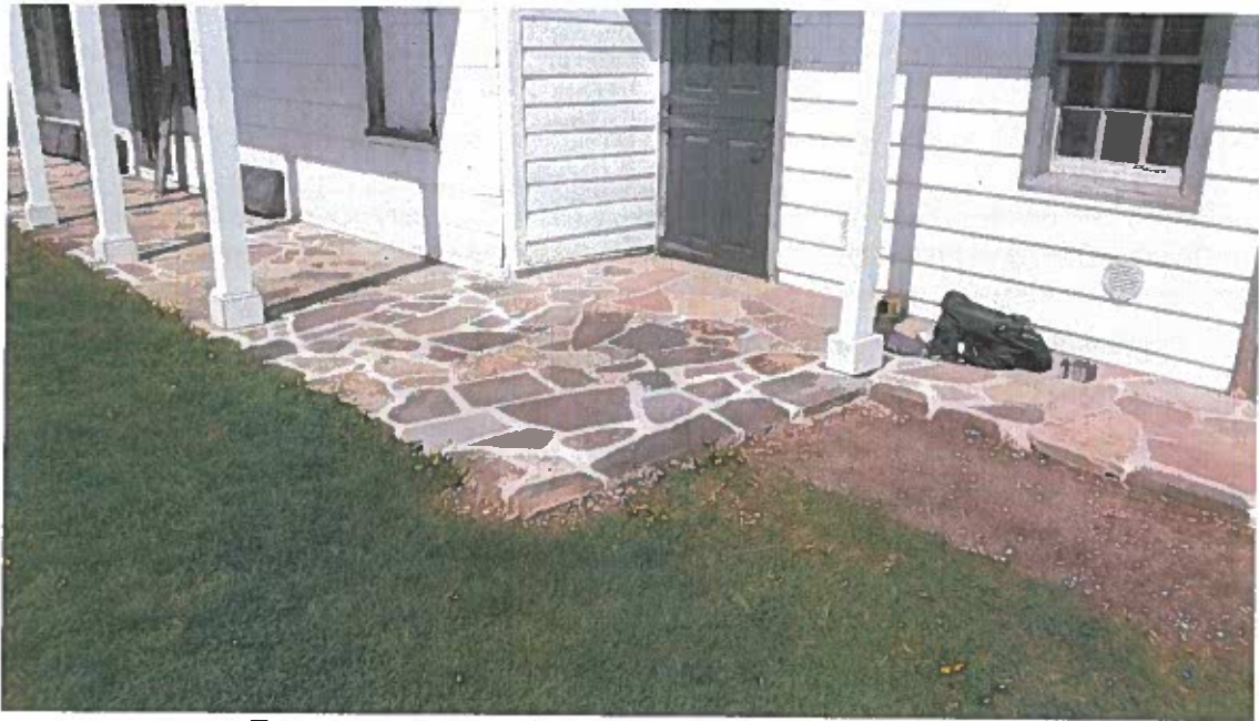
Entrance to Rockingham House requiring ADA access.
