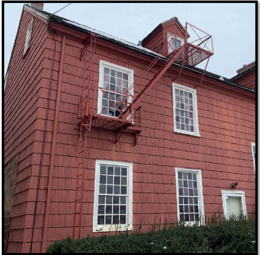
Photograph From Fire Escape Repairs
