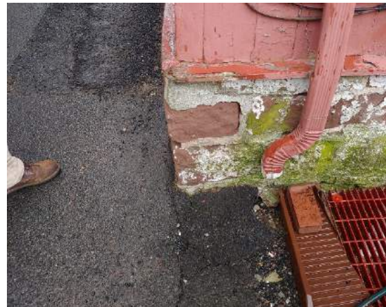
Northeast Building Corner Photograph 7
