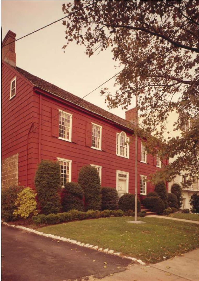
Plate 3.2: Overview of the project location showing the paved driveway to the west (left), areas of landscaped plantings, and the rainwater drainage gutter running from the roof toward the ground surface.
