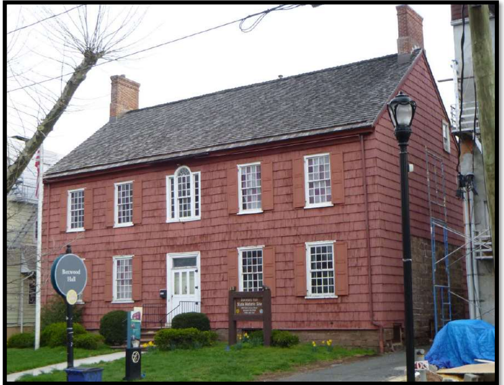
New Roof Installed at Boxwood Hall Residence
