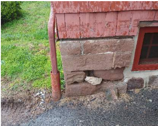
Southeast Building Corner Photograph 6
