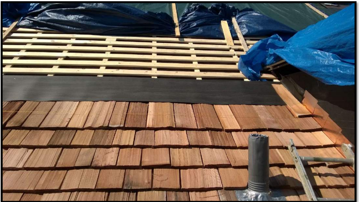
Photograph Taken During Roof Replacement
