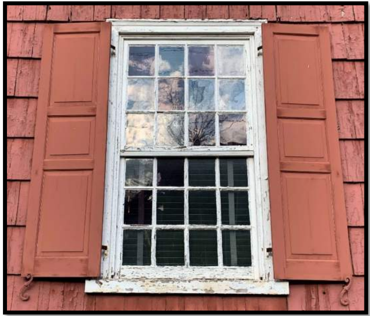
Overall View of North Facade Window
