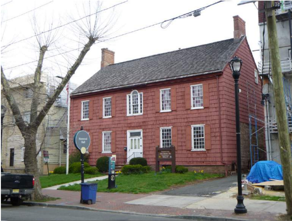
Plate 4.1: Overview of the Boxwood Hall building taken from the south side of East Jersey Street.
