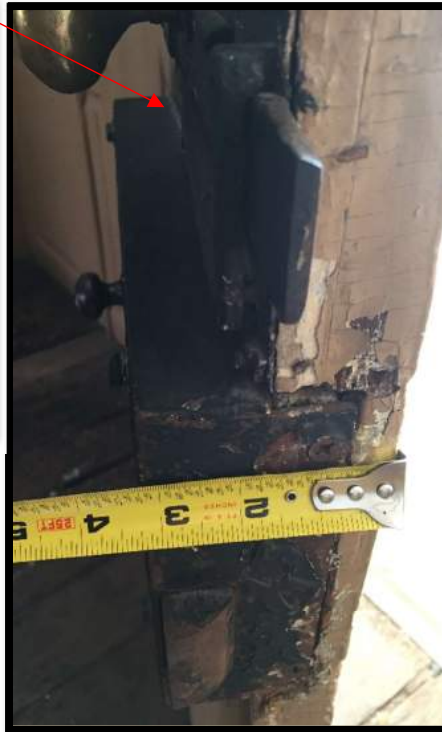
Crack in Bottom Sill
