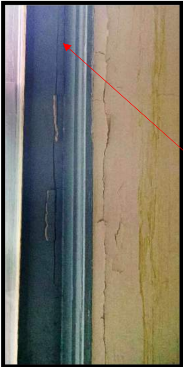
Cracking Around Interior Wood Trim
