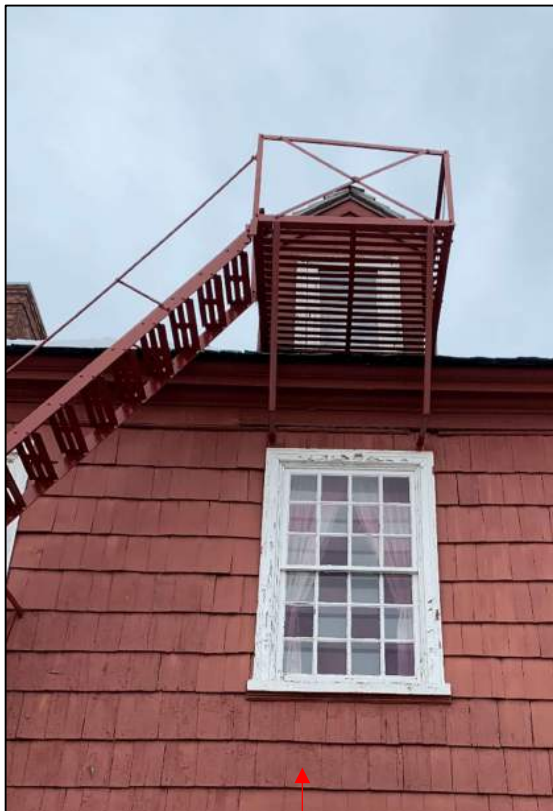
Overview of Emergency Egress Above Window
