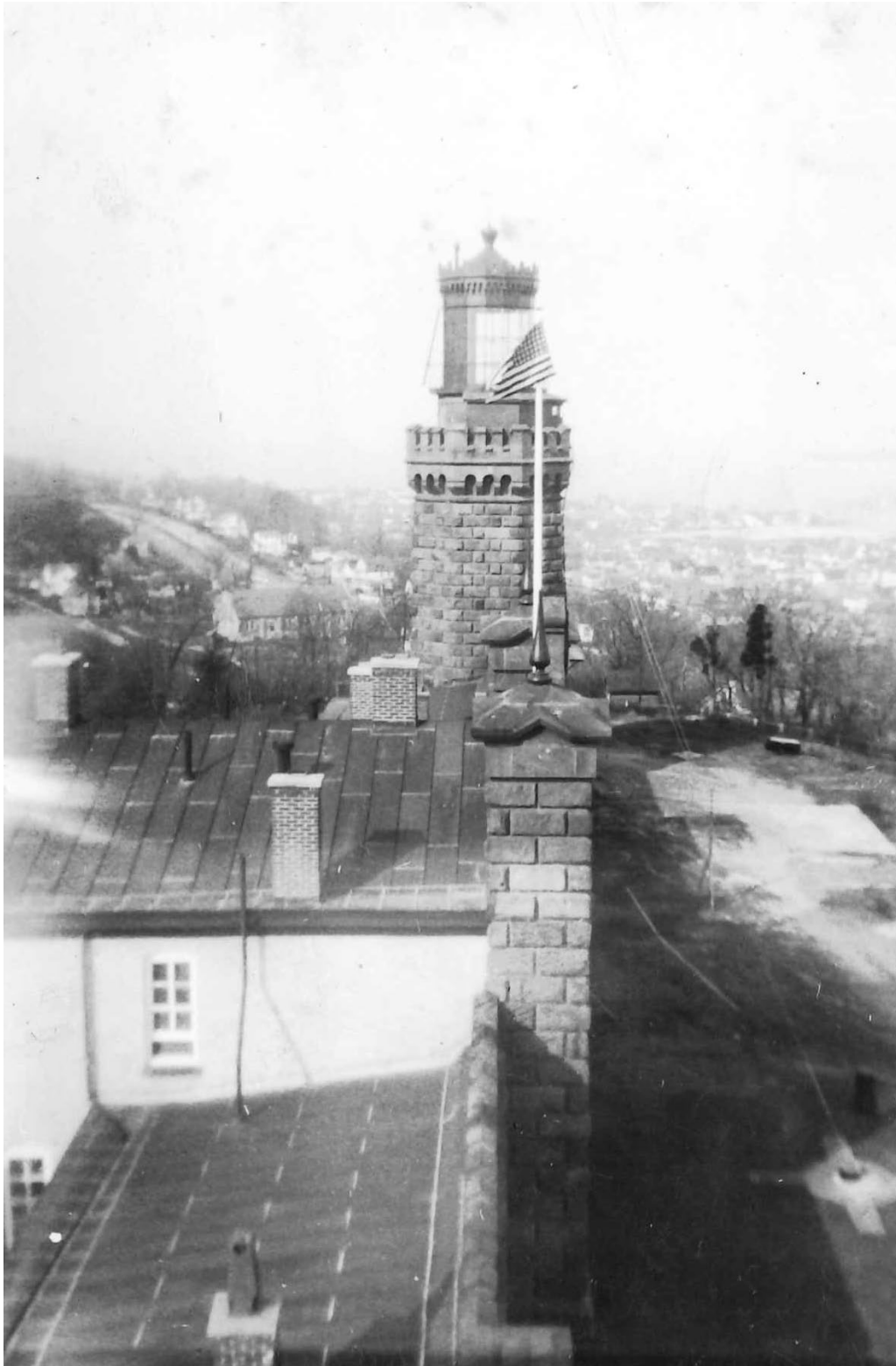
1945 – Roofing Close-up prior to Lighthouse closure & pre-restoration
