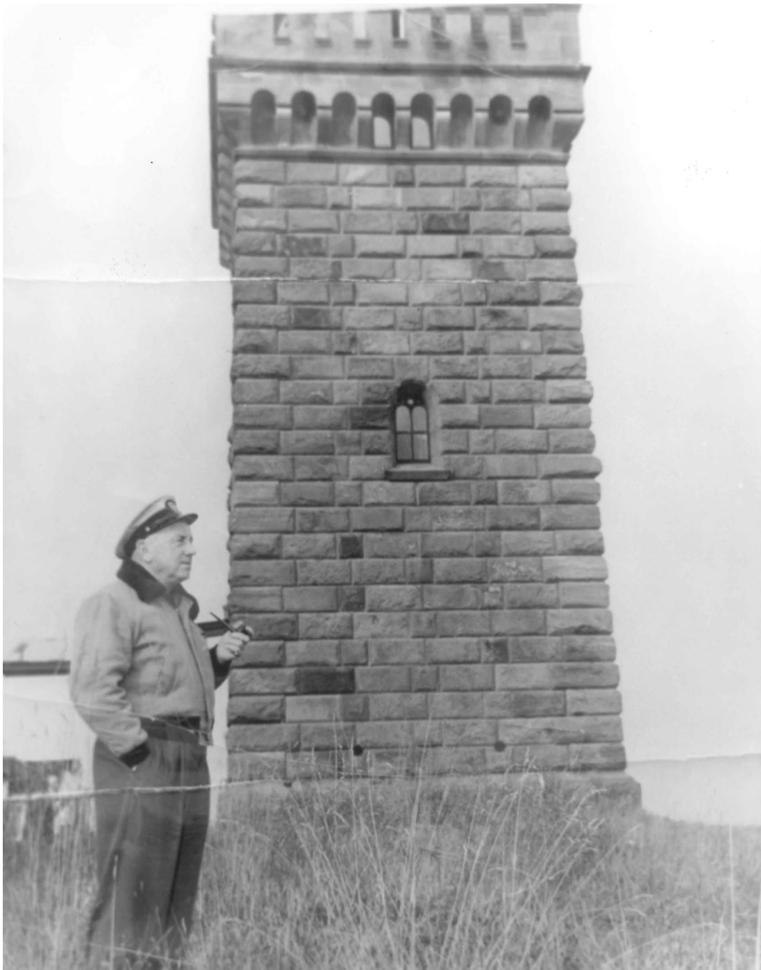
Figure 6: ca. 1940 Keeper Murphy Rockette posing with the South Tower. Note that the tower window trim is brown.
