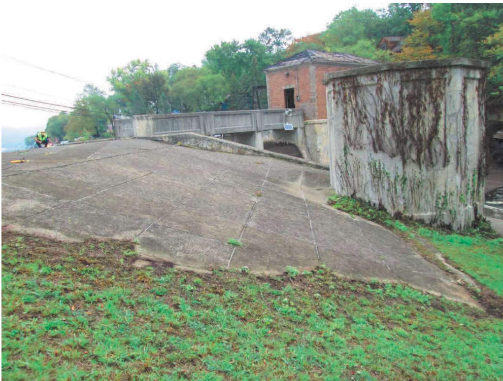
Photo No. 12: Concrete paving along the upper downstream slope above the surge tank looking left.
