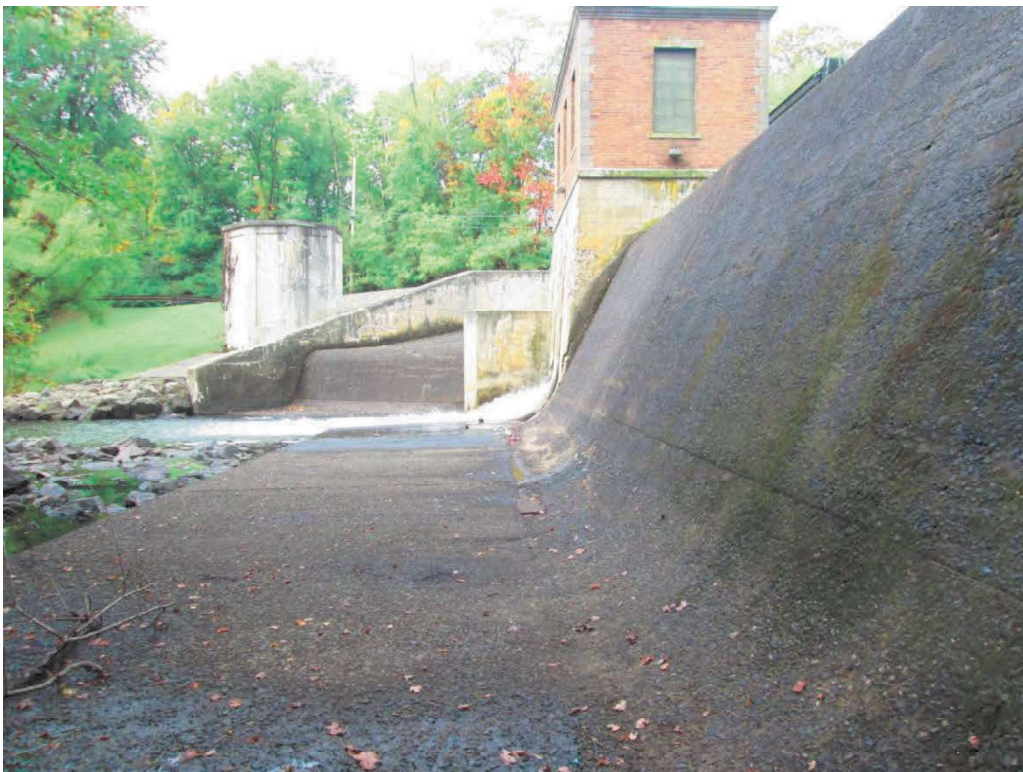
Photo No. 30: Downstream face and apron of the 90-foot long spillway weir looking right.
