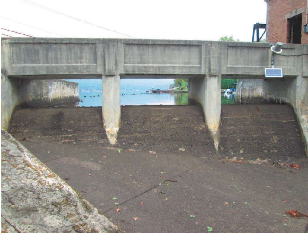
Photo No. 21: Crest and downstream face of the 30-foot long spillway weir looking upstream.
