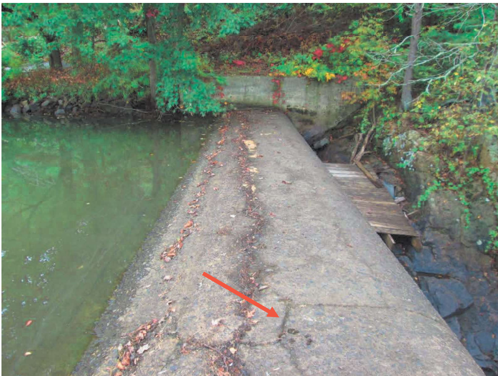
Photo No. 28: Crest of the 90-foot long spillway weir looking left. Note the left keyway joint.
