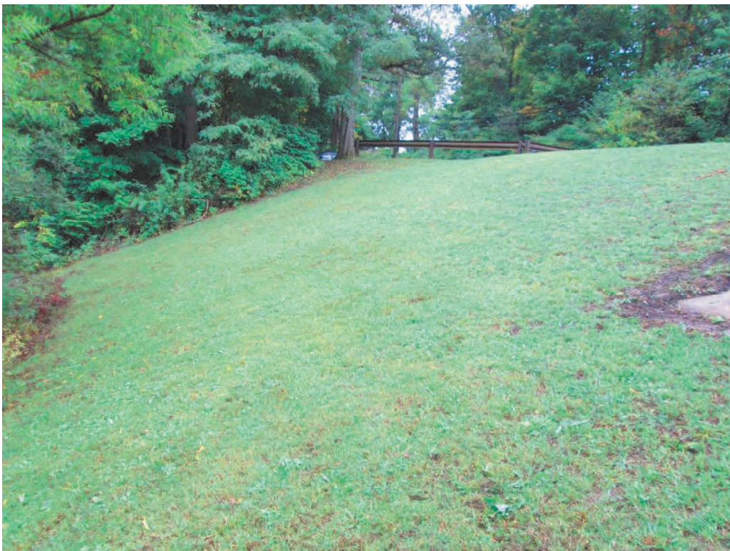
Photo No. 10: Cellular concrete block mats (covered by grass) on the downstream slope of dam looking right.
