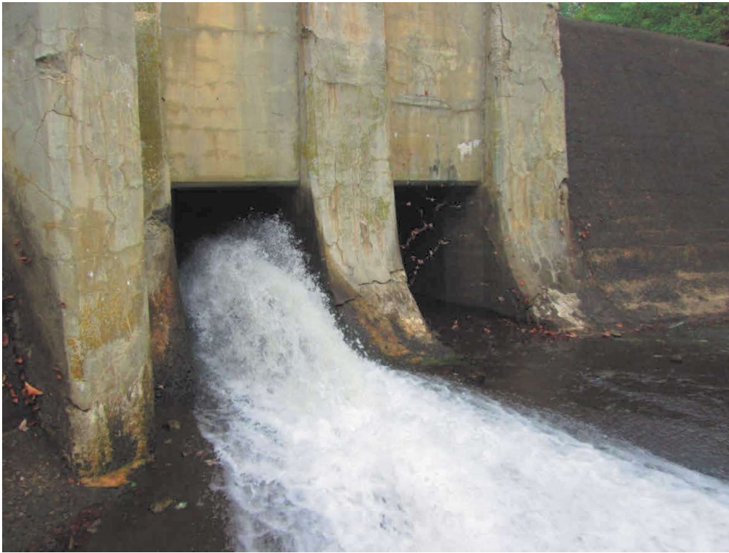
Photo No. 43: Downstream side of the gatehouse and low level outlets.
