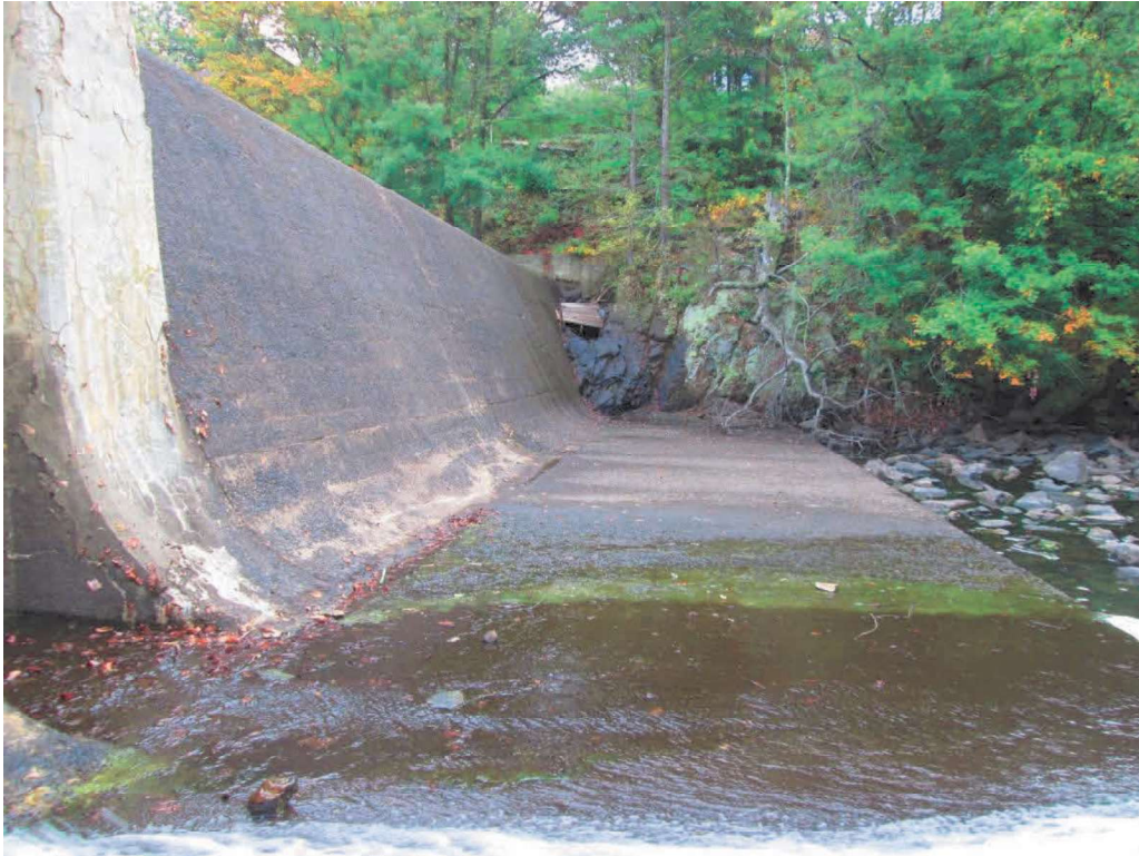
Photo No. 29: Downstream face and apron of the 90-foot long spillway weir looking left.
