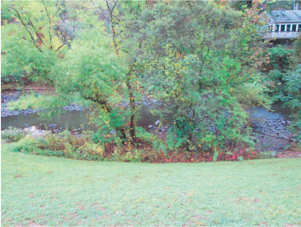
Photo No. 9: Cellular concrete block mats (covered by grass) on the right side downstream slope of dam looking downstream.
