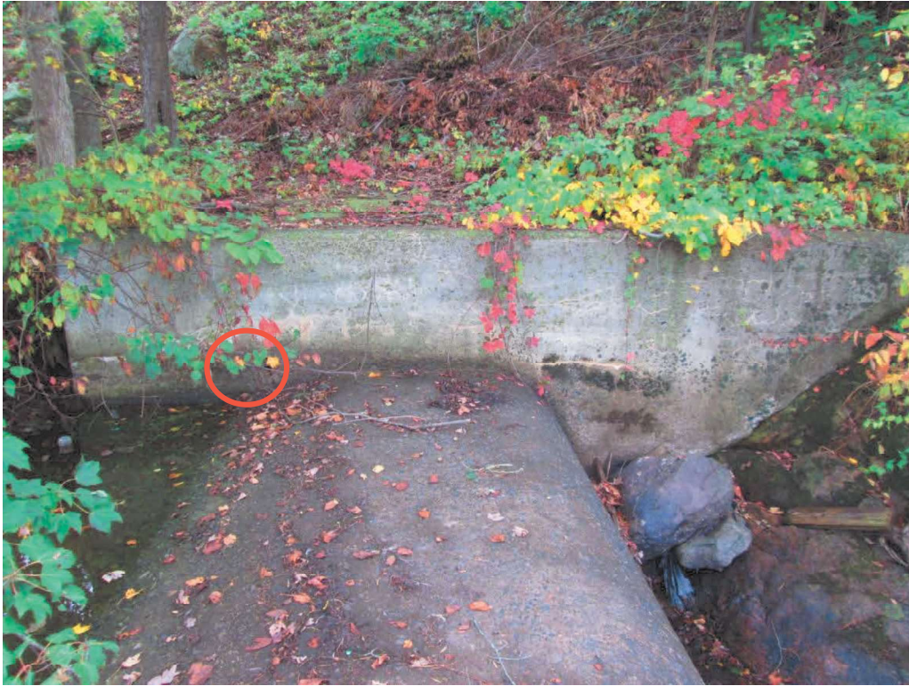
Photo No. 35: Left training wall at the contact with the 90-foot long spillway crest and left abutment. Note the location of the small void in the training wall.
