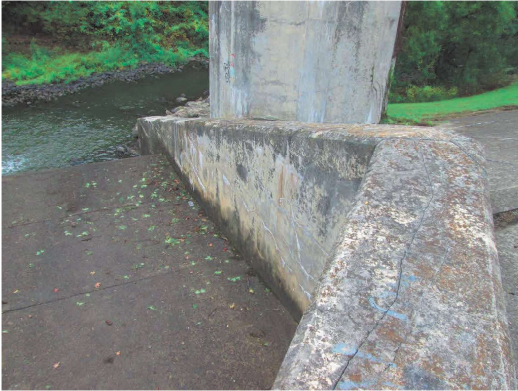
Photo No. 23: Downstream right wing wall at the 30-foot long spillway weir looking downstream.
