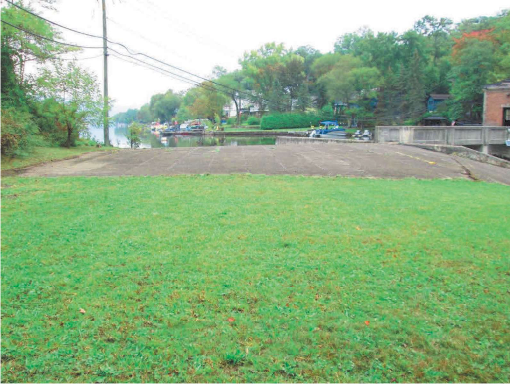
Photo No. 3: Cellular concrete block mats (covered by grass) and concrete paving sections of the dam crest looking upstream.
