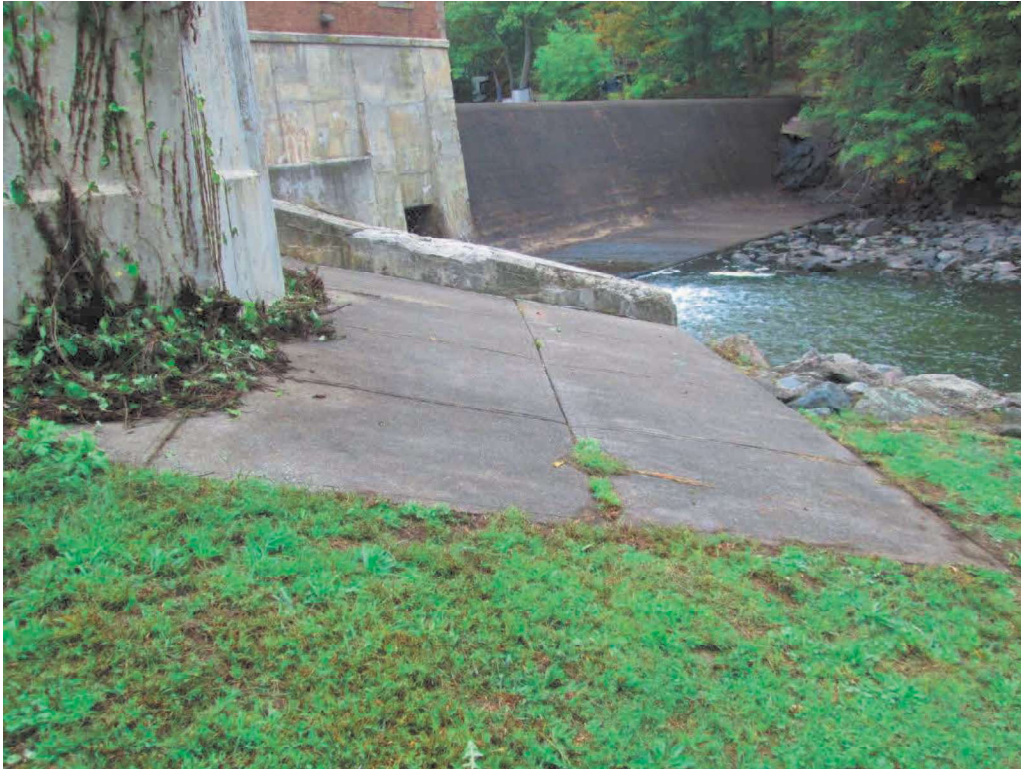
Photo No. 15: Concrete paving along the lower downstream slope below the surge tank looking left.
