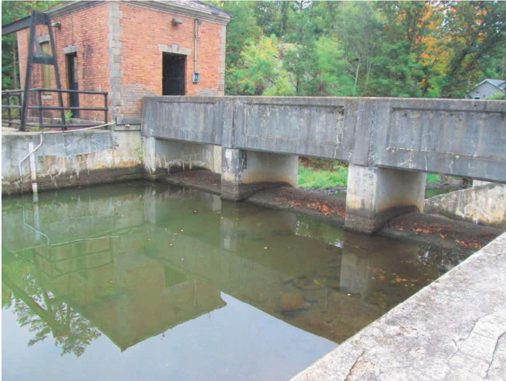
Photo No. 19: Entrance channel to the 30-foot long spillway weir looking downstream.
