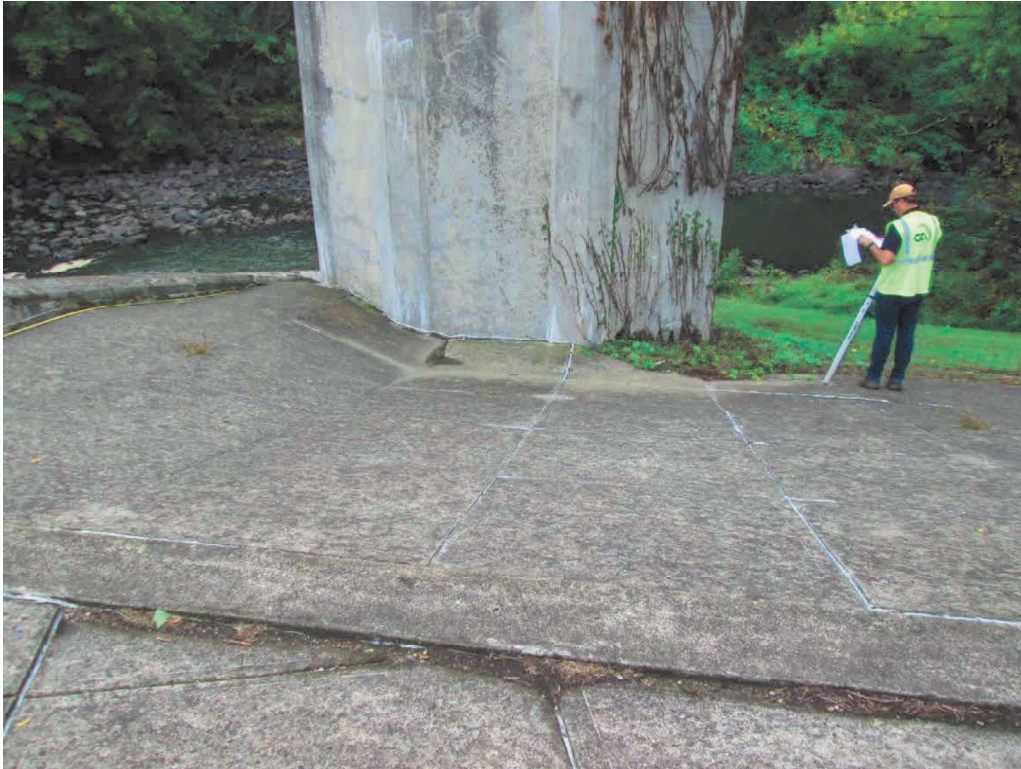
Photo No. 13: Concrete paving on the downstream slope at the contact with the upstream face of the surge tank looking downstream. Note the vines growing on the surge tank.
