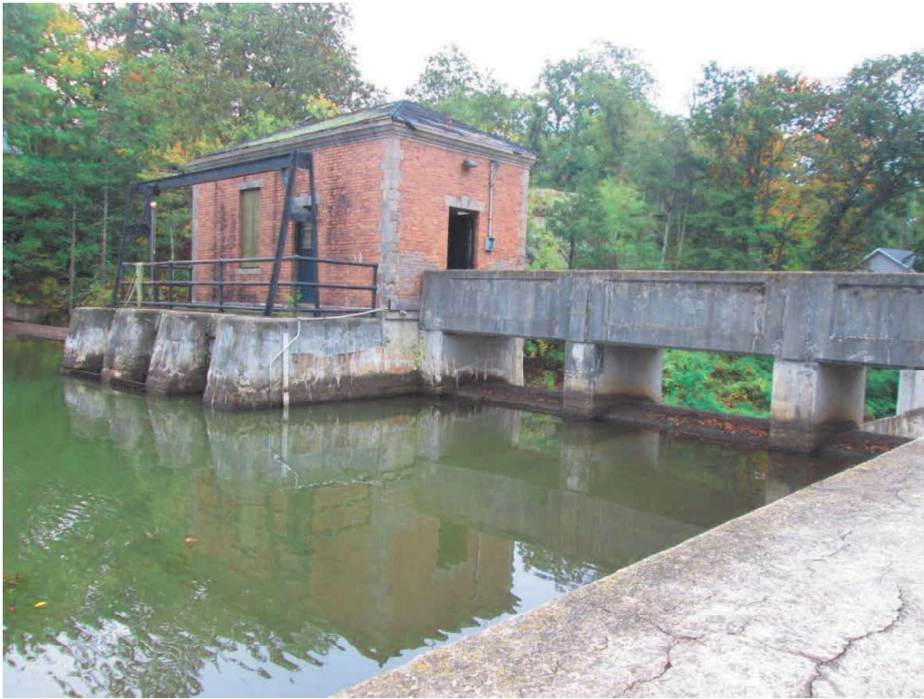
Photo No. 41: Gatehouse and low level outlet entrance.
