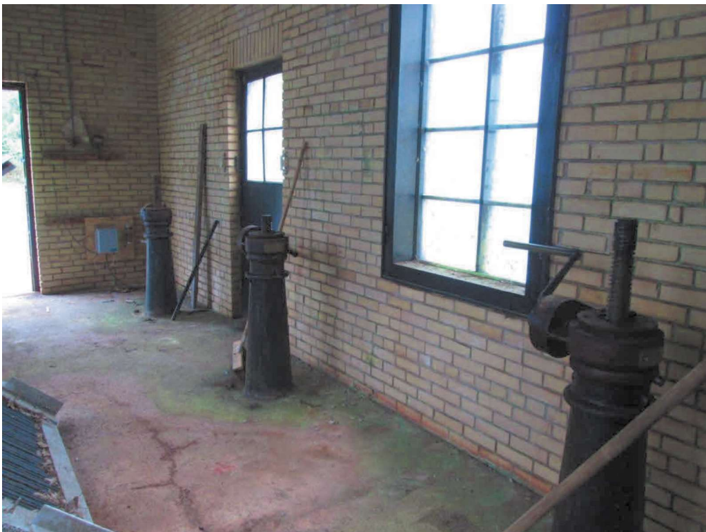
Photo No. 42: Interior of gatehouse and the hand crank operators for the sluice gates.
