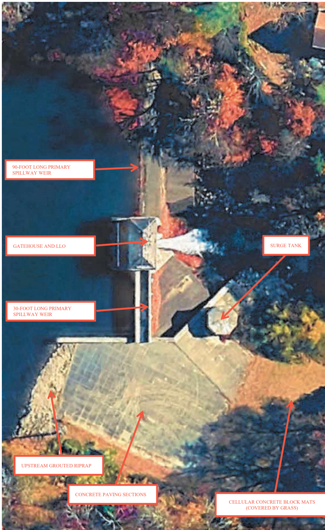
Aerial view of Greenwood Lake Dam.
