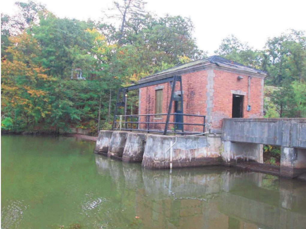
Photo No. 25: Entrance channel of the 90-foot long spillway weir looking left.
