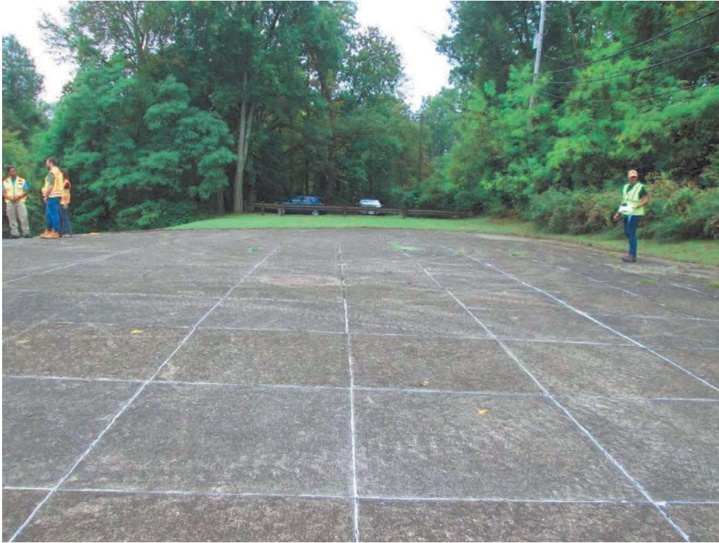
Photo No. 1: Concrete paving sections of the dam crest looking downstream.
