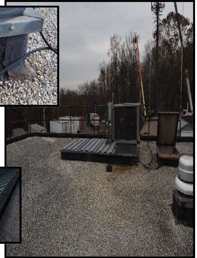
Built-up Roofing System
