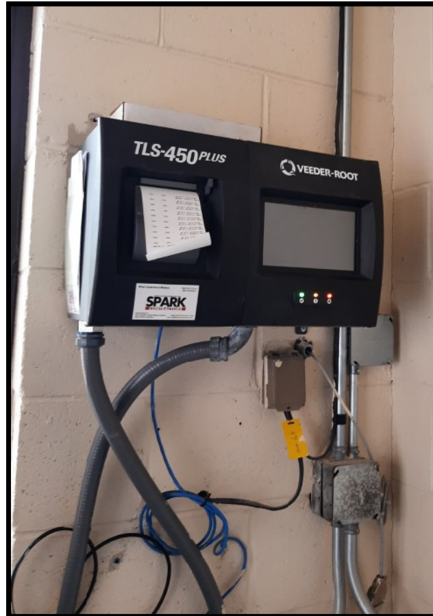
Existing Veeder Root Tank Measurement Controls
