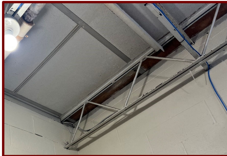
Existing Roof Structure at Academic Center
