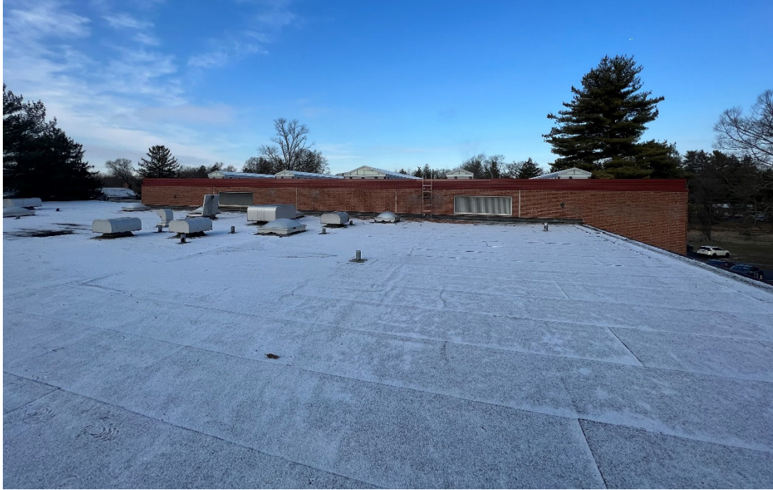
Overview of Roof and Proposed HVAC Unit Location
