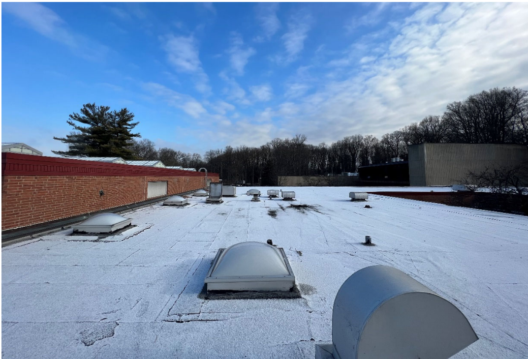
Overview of Roof and Proposed HVAC Unit Location
