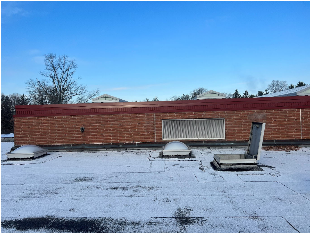
Existing Exhaust Ventilation Penetration at Gymnasium Roof
