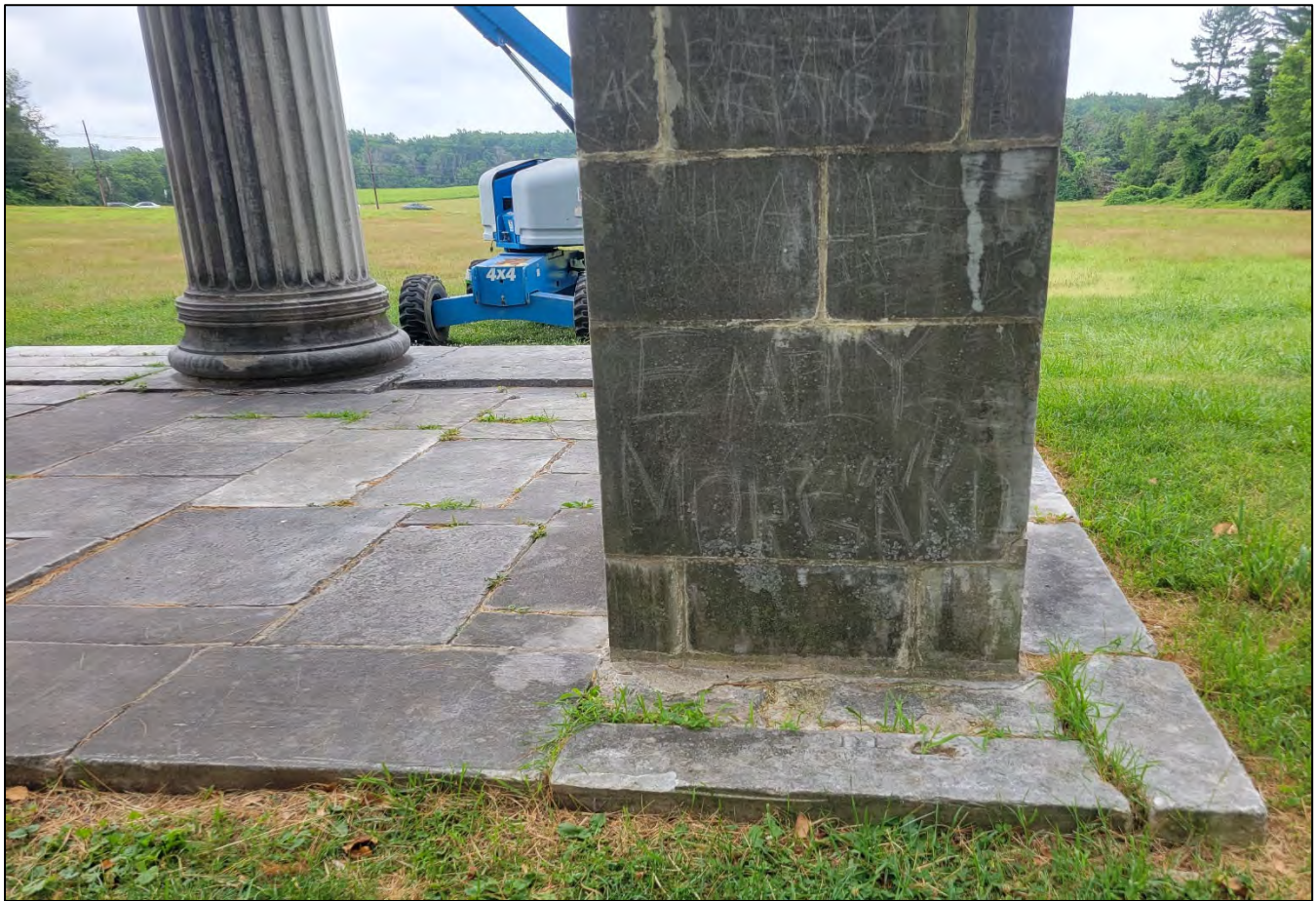
Photo 17: Detail of the paving behind the piers showing general conditions. The stones at this location differ from the others being generally smaller and less regular in shape. The scratched graffiti is pronounced at the rear of the piers but was observed at other locations as well. The unevenness of the pavers is clearly visible.
