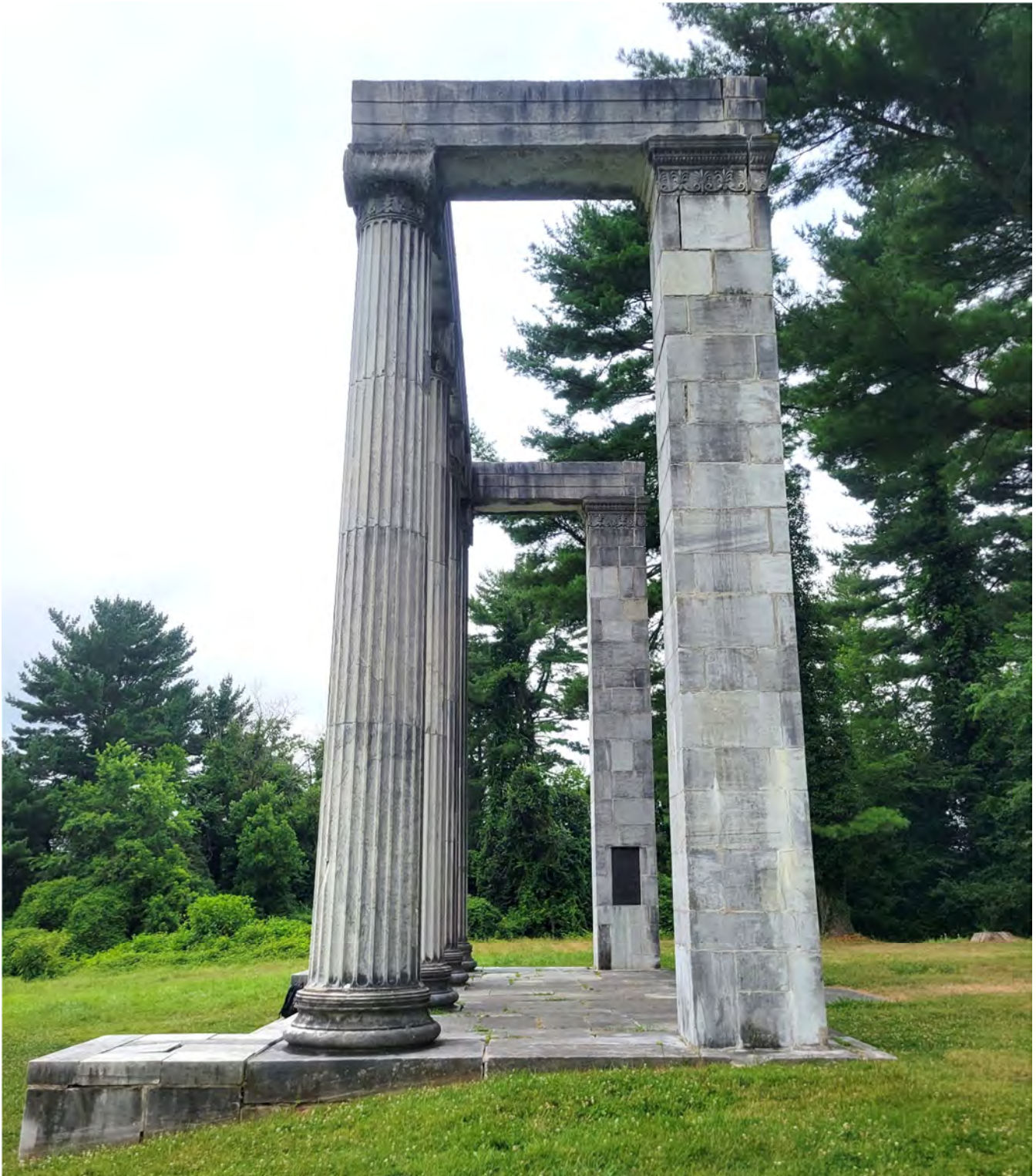
Photo 3: View of the east elevation showing the shape of the structure and the stair cheekwalls and marble pavement.
