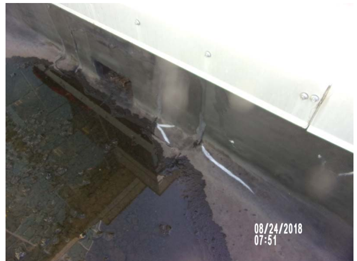
3. Typical opening in corner patch.
