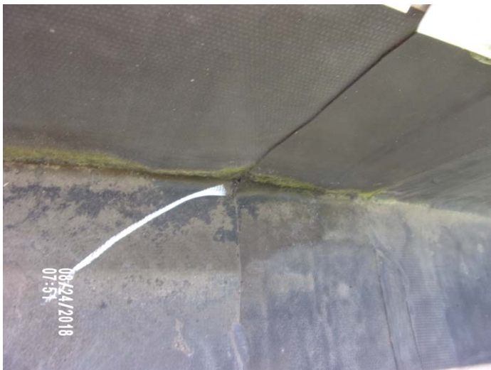
3. Typical opening in corner patch.
