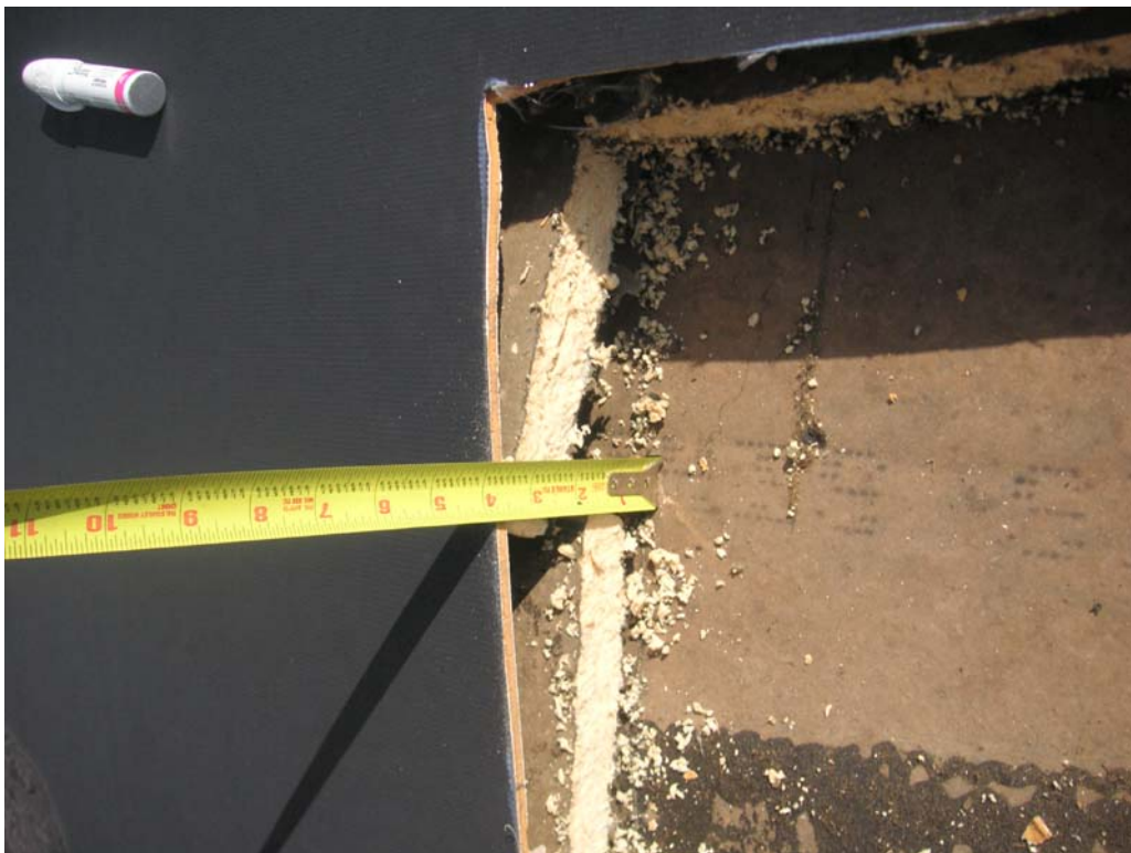
35. 4" rise of membrane and hard board
