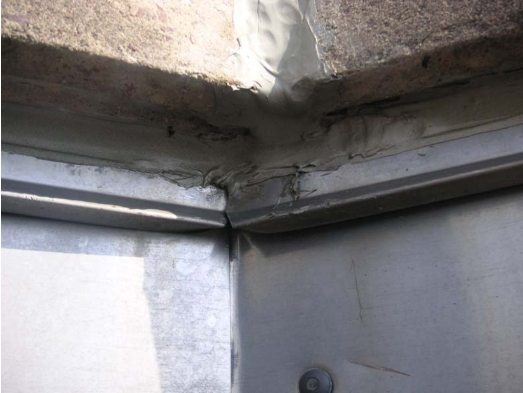
52. Leakage point for wall systems
