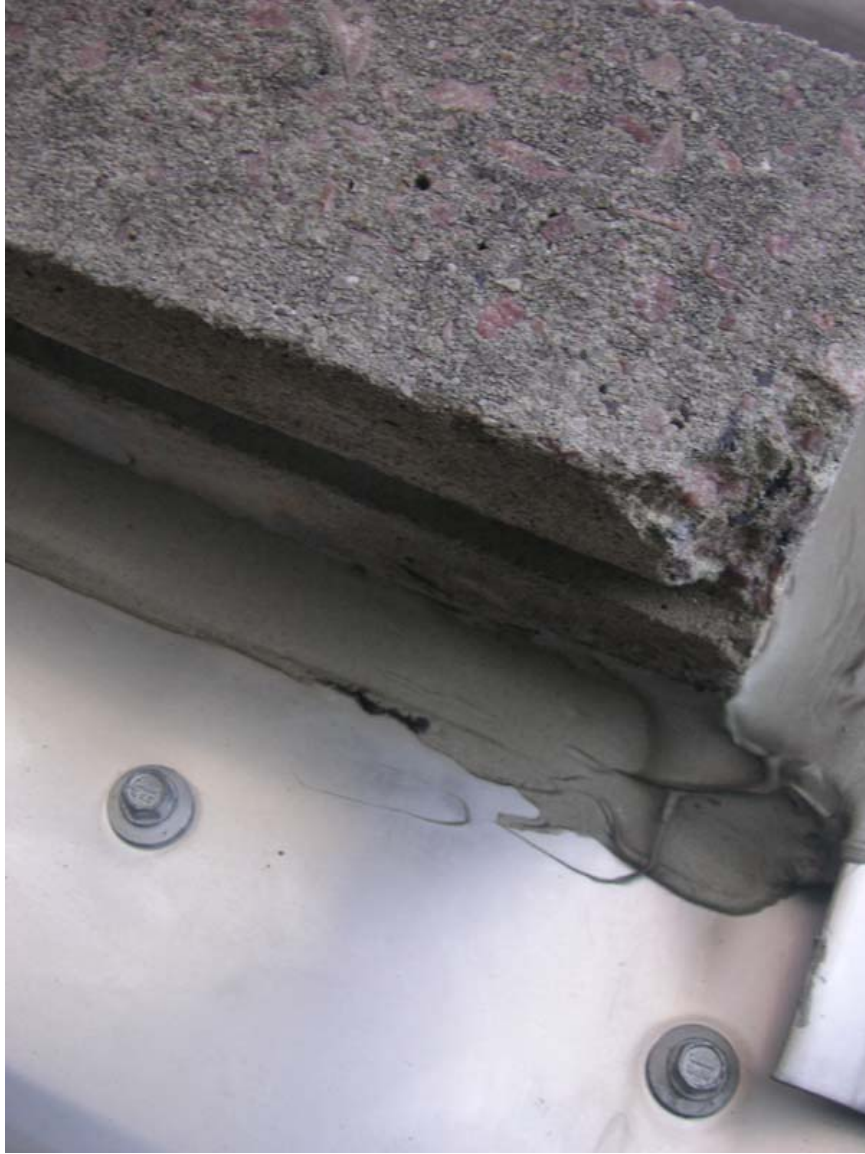
45. Caulk joint at crenel section
