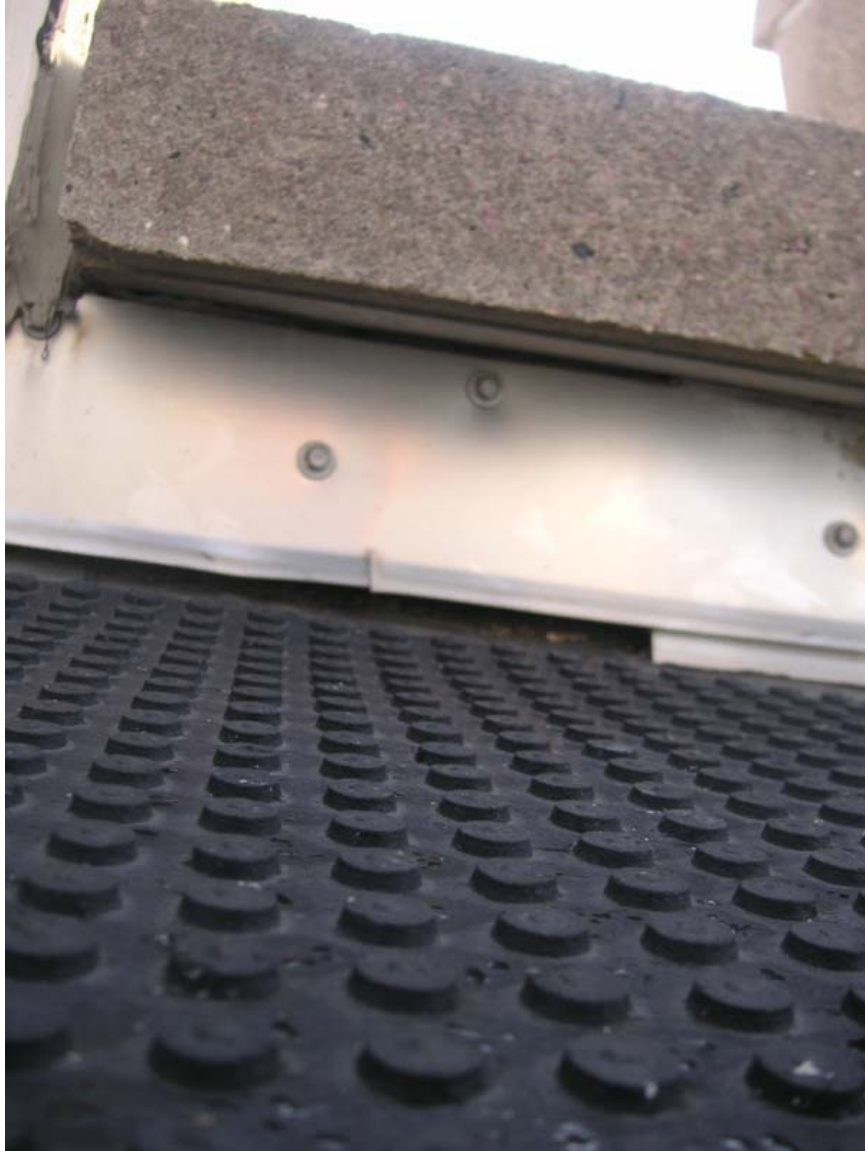
44. View of counterflashing detail at bottom of crenel
