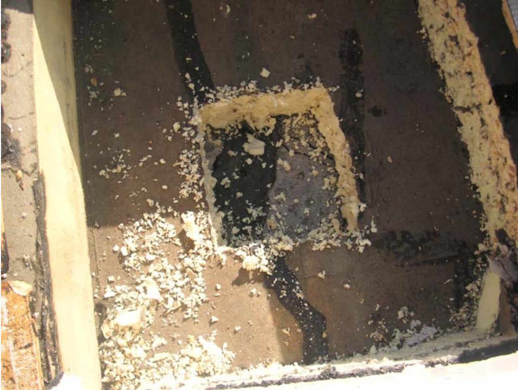
23. Base layer cut away; good attachment to concrete substrate
