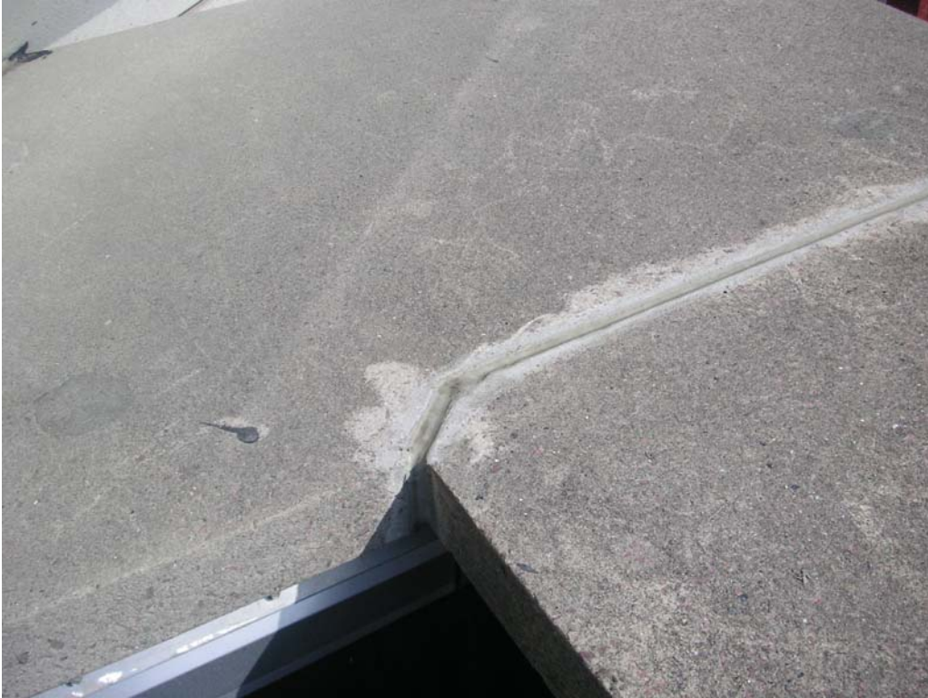
46. Top of caulking for cast stone
