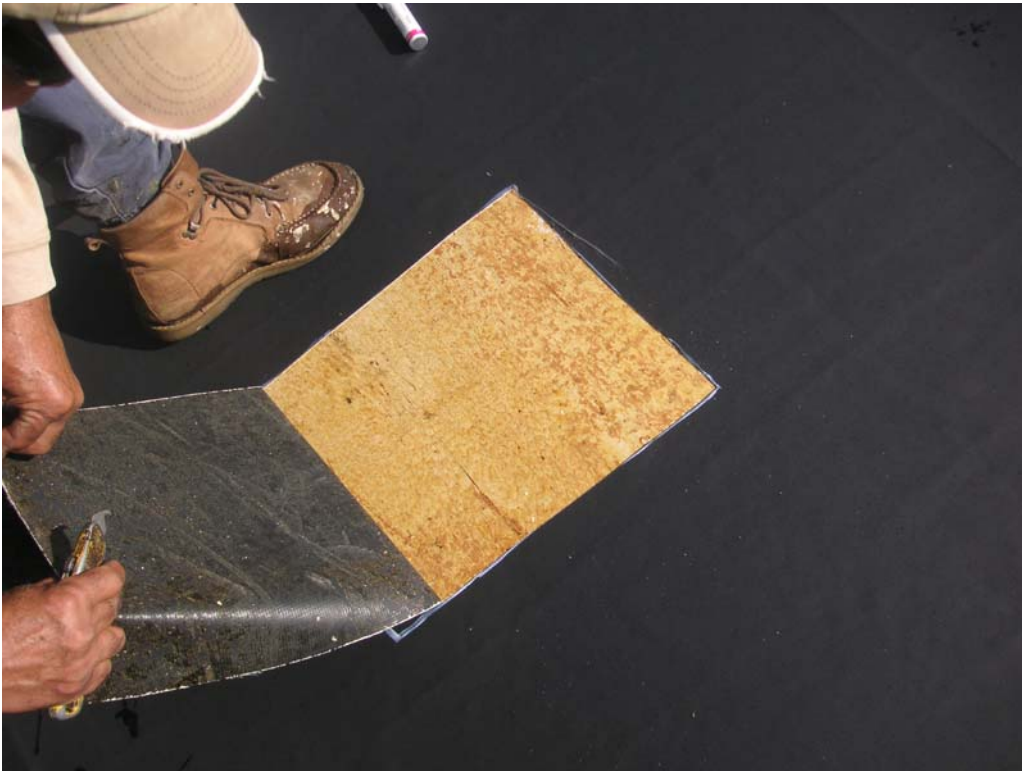
29. Good attachment of membrane to hard board
