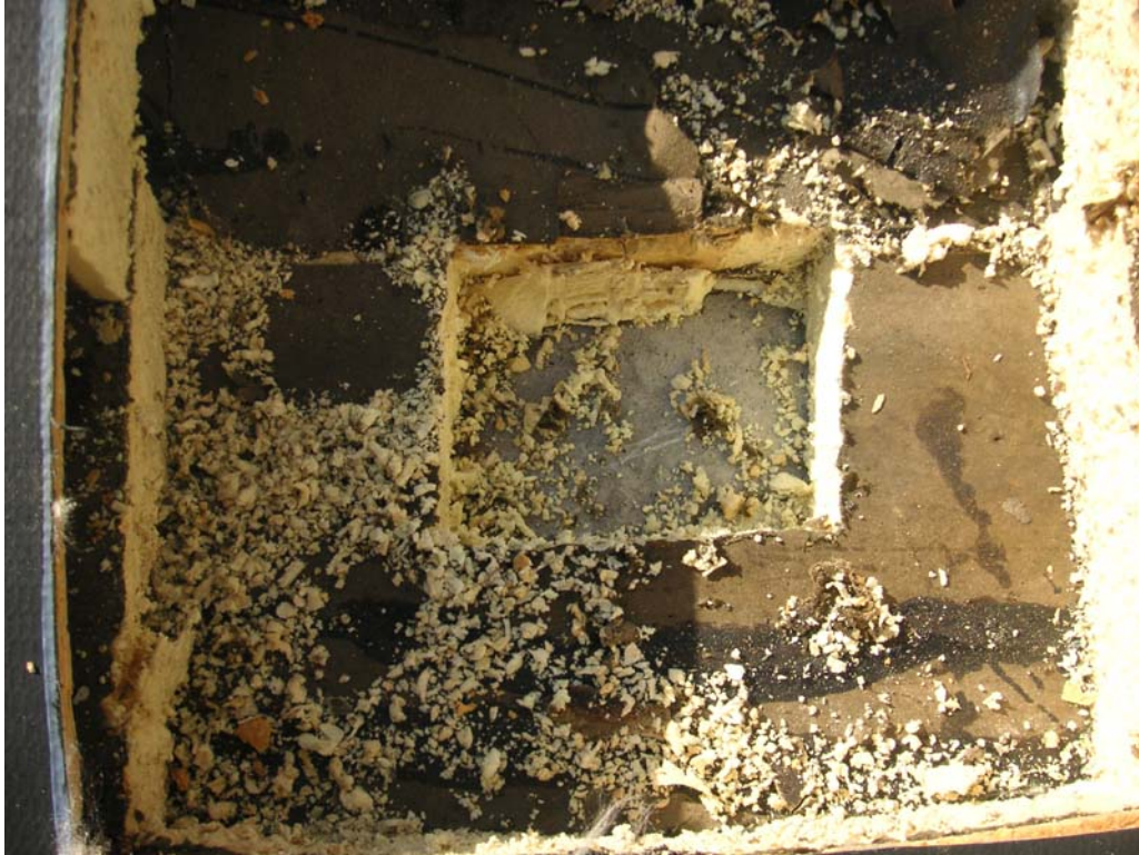
7. Bottom layer removed to concrete deck
