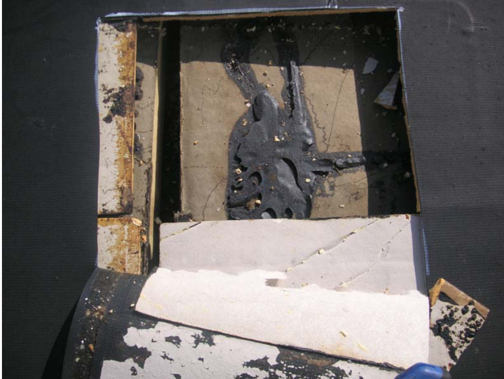
19. Good attachment of hard board to insulation
