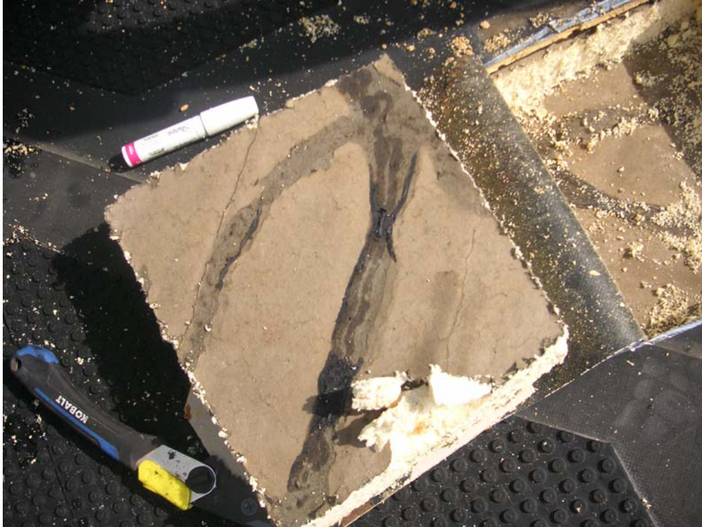
68. Shear top board of insulation
