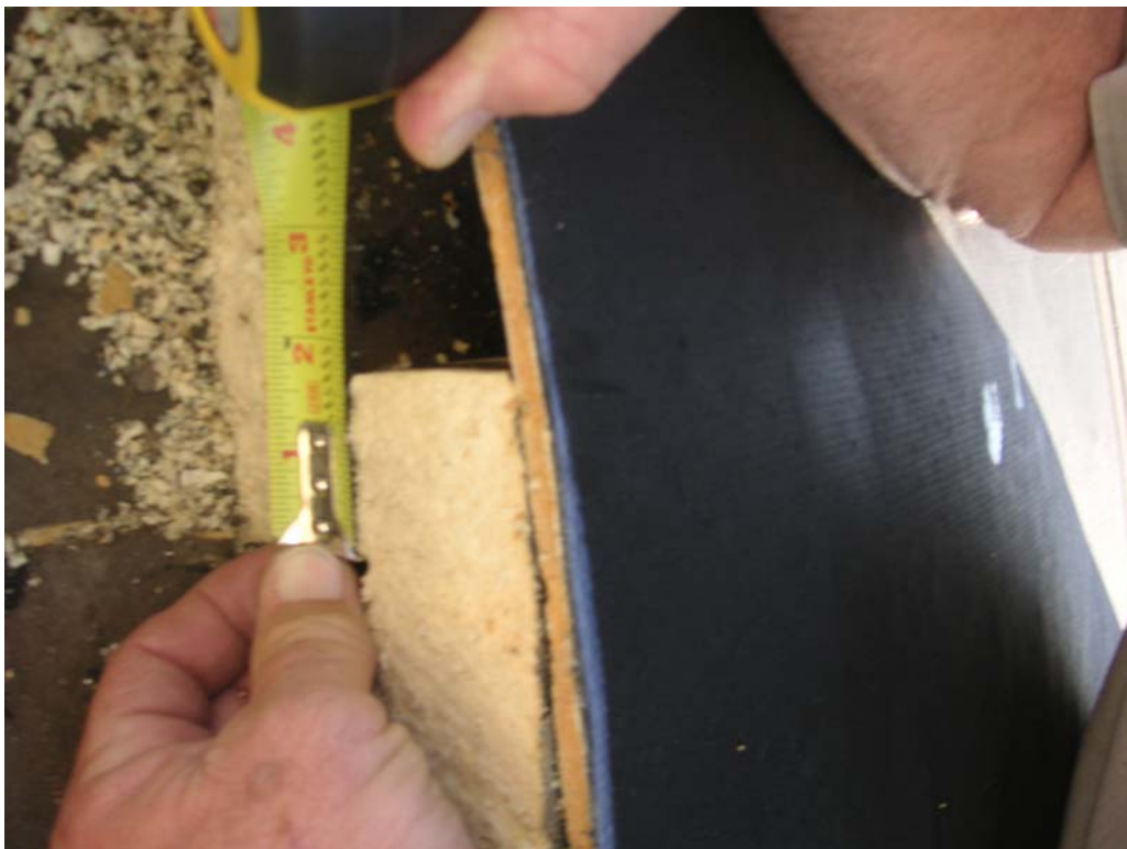
8. 1.5" overlay of board; board is juxtaposed to adjacent board
