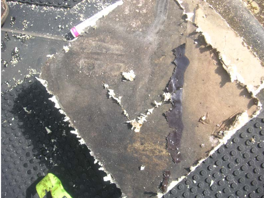
70. Underside of bottom layer of board
