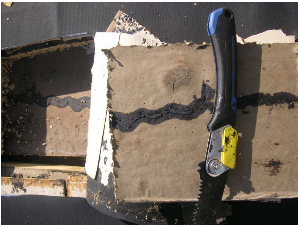
20. Top layer removed; good attachment to base board
