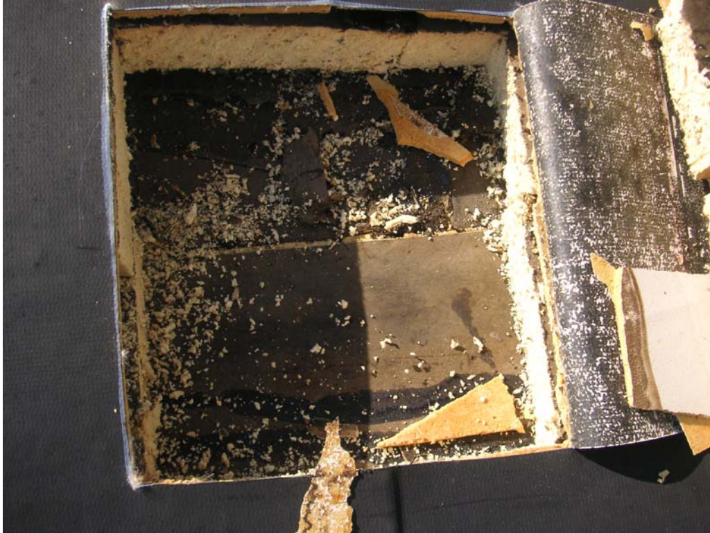
5. Bottom layer to concrete deck
