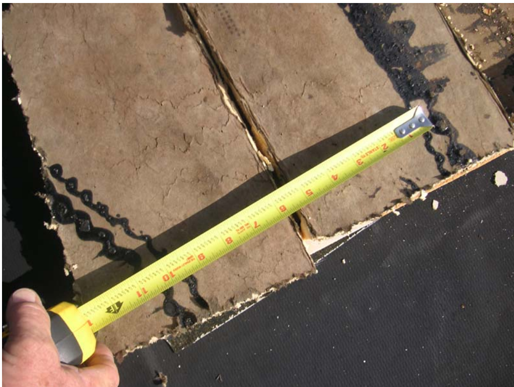
33. Full attachment as to manufacturer's recommendations at 10" for interface
