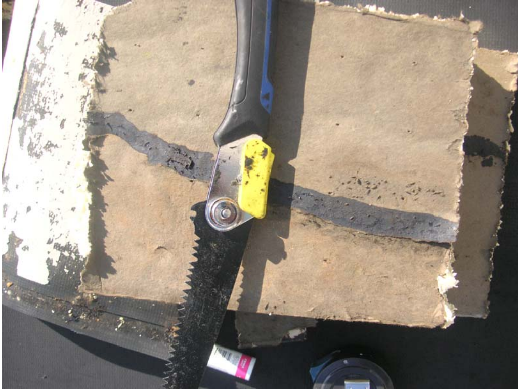
21. Underside of top layer
