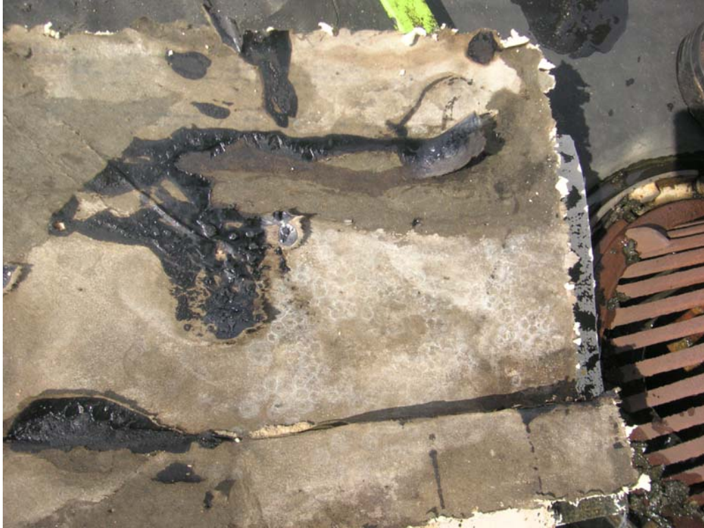
88. Mold spores bottom of 1st board
