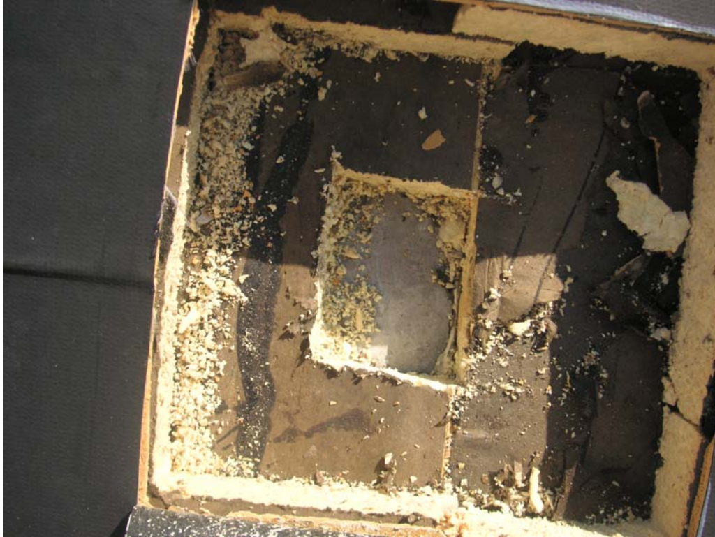
13. Good attachment of insulation to insulation interface
