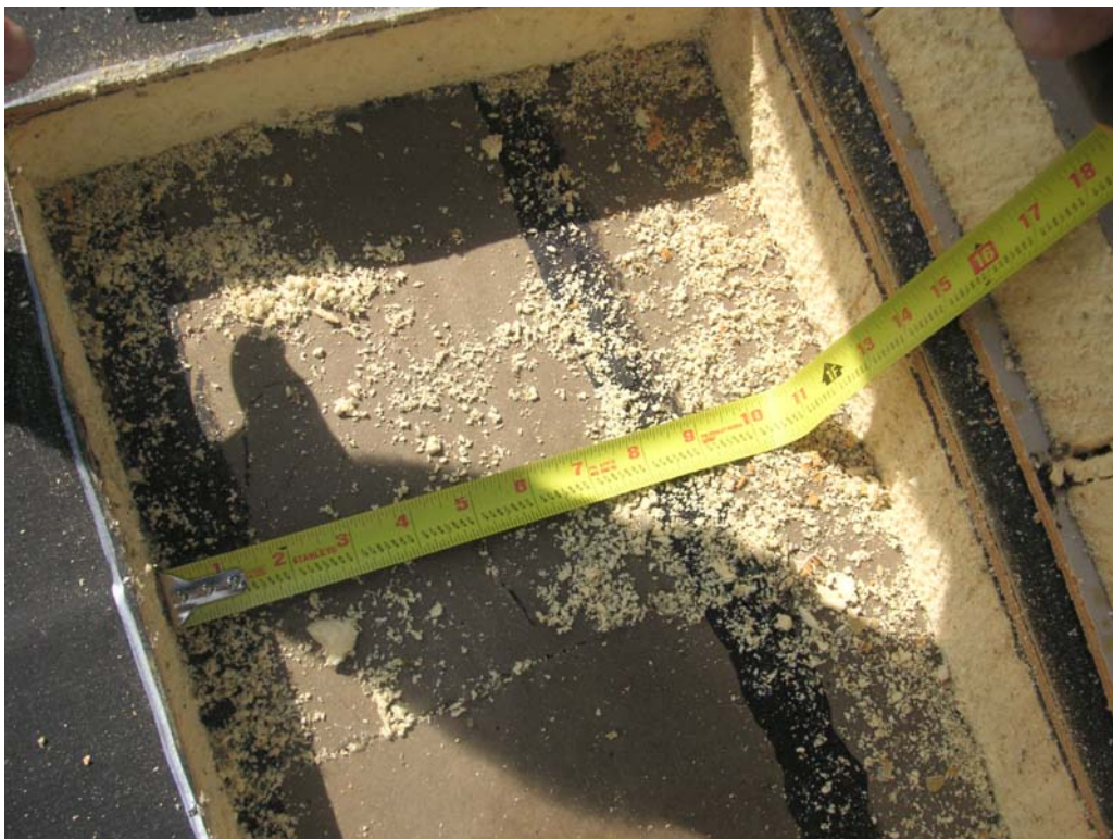
79. Good attachment of insulation layers
