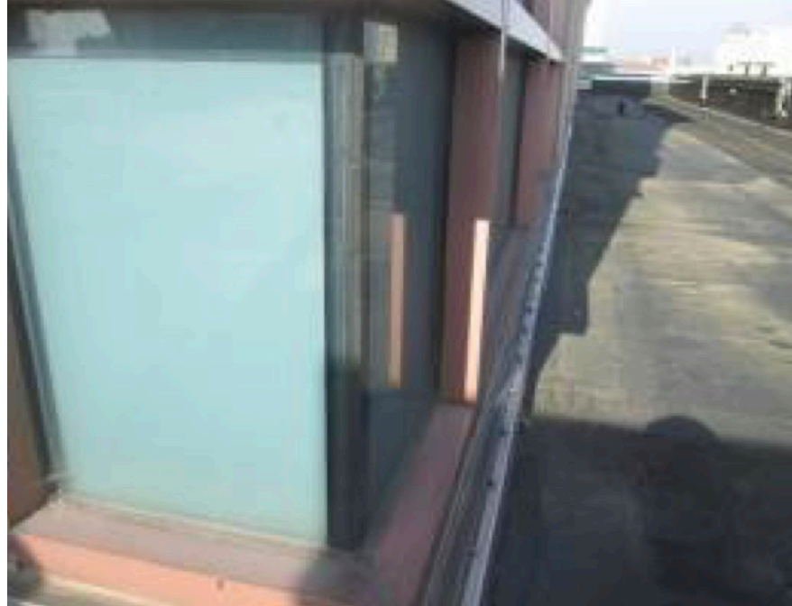
9. Caulking at Windows.
