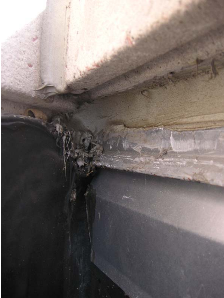
47. Caulking above cast stone and counterflashing
