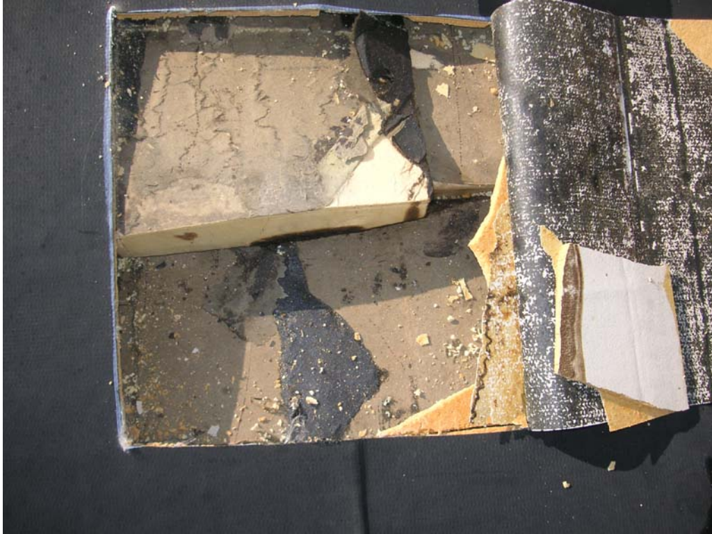
3. Top layer of insulation riding over the adjacent layer
