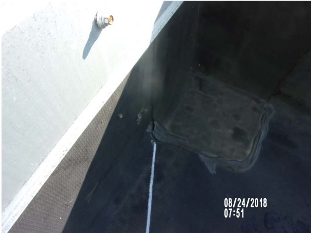
3. Typical opening in corner patch.
