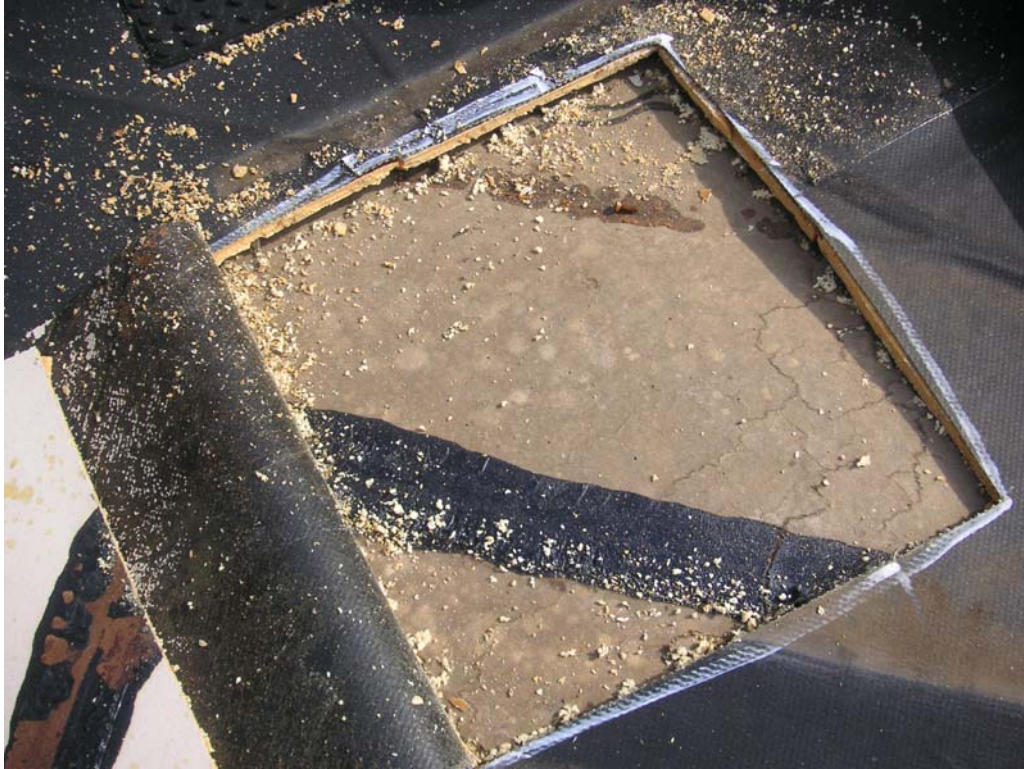
66. Good attachment of hard board; note mold spores
