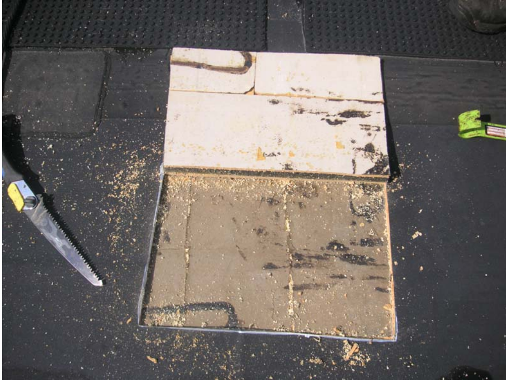
76. Attachment of hard board to base insulation
