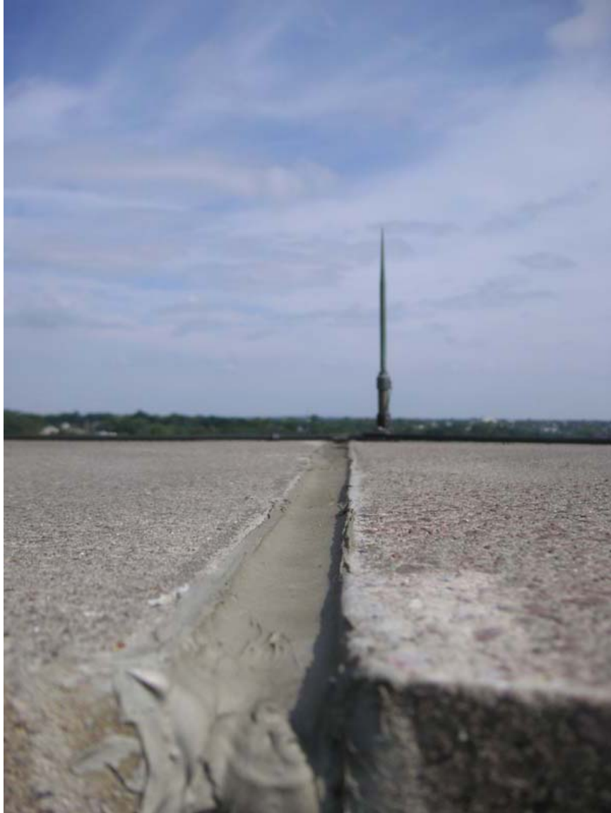
51. Top re-facing of stone for caulk
