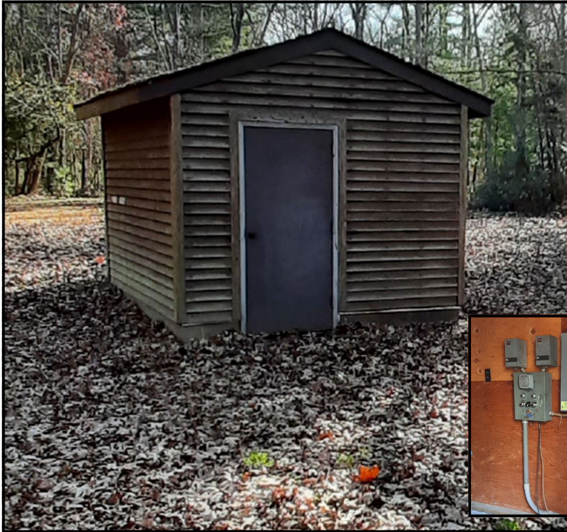
Water Pump Shed
