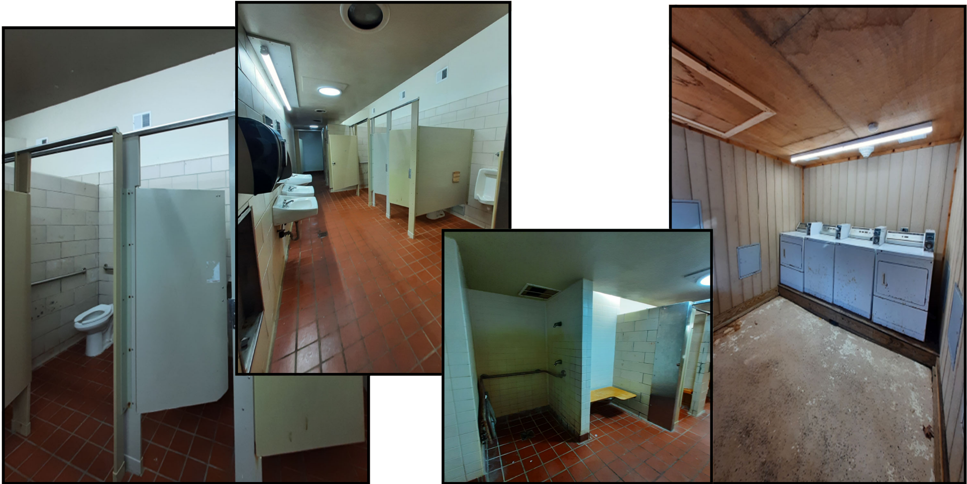
Combined Toilet & Shower Room
