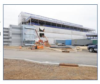
head service carriers were being installed and laboratory casework deliveries had commenced. The exterior wall systems were completed by year end with the exception of the Administrative Wing area. Also during 2009, construction of the Pre-Screening Building and the Greenhouse commenced.
