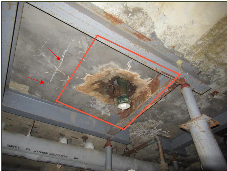
Photo No. 8 – Cracked and spalled concrete slab underside (below trench drain)
