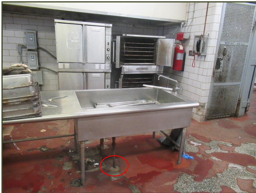
Photo No. 6- Open holes surrounding kitchen sink drain.
