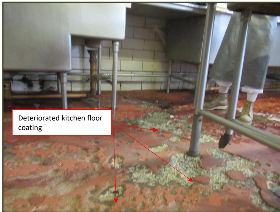
Photo No. 3 – Typical deteriorated kitchen floor coating
