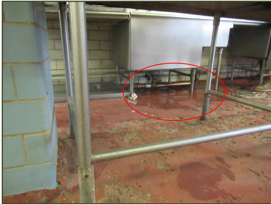
Photo No. 7 – Ponding soap water below sink
