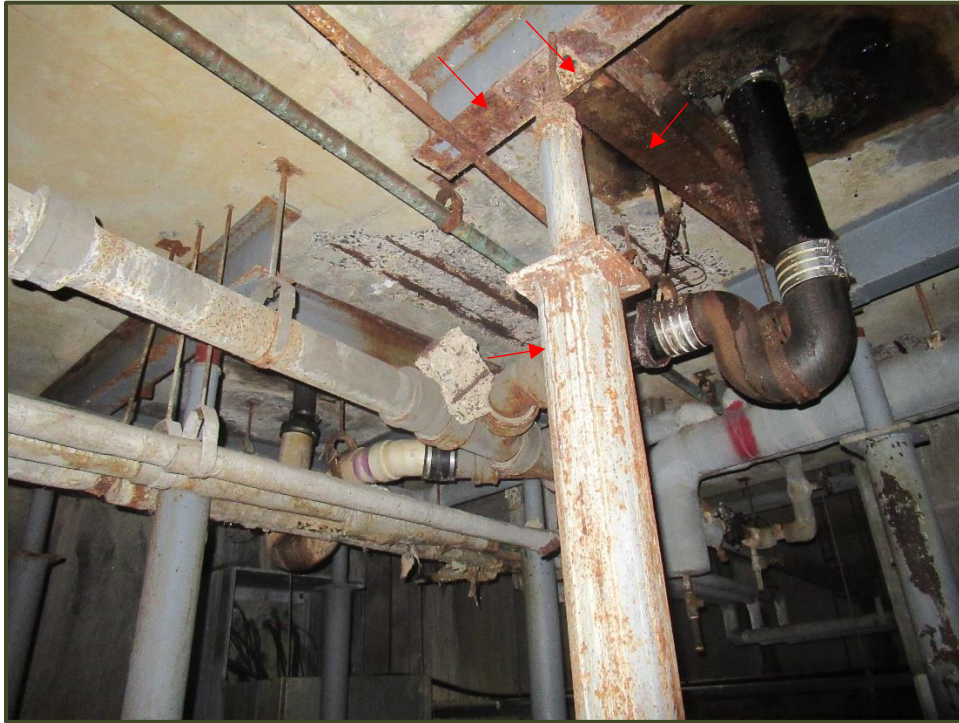
Photo No. 9 – Corroded shoring beams and posts
