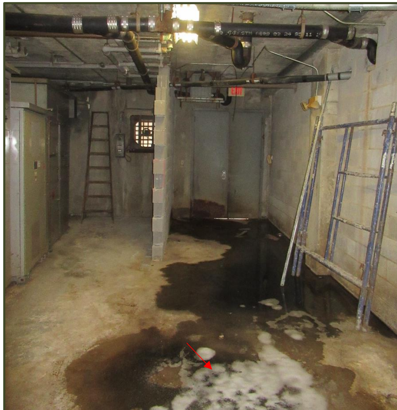
Photo No. 12 – Ponding water below kitchen sink drain
