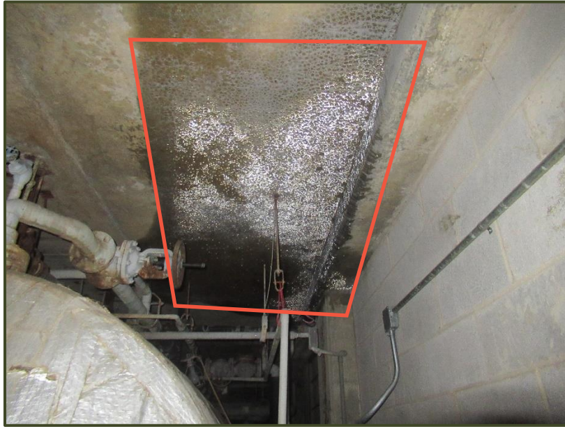
Photo No. 11 – Active water staining at the underside of the concrete slab
