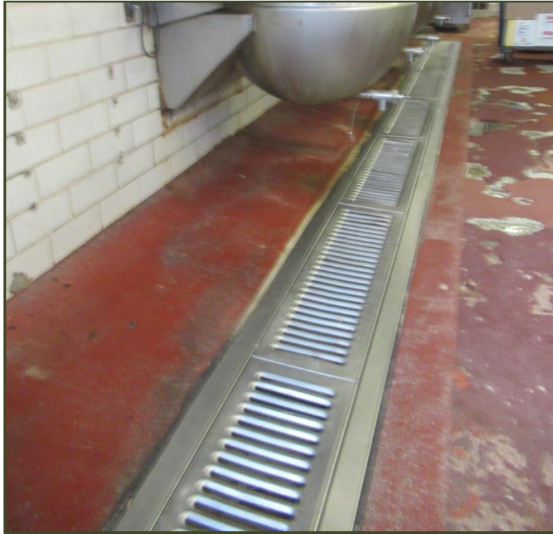
Photo No. 5- Existing Kitchen Trench Drain
